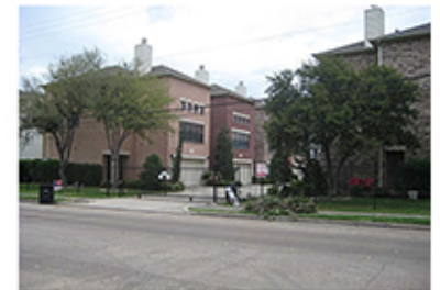
TOWNHOME DEVELOPMENT ACROSS THE STREET FROM SUBJECT SITE
