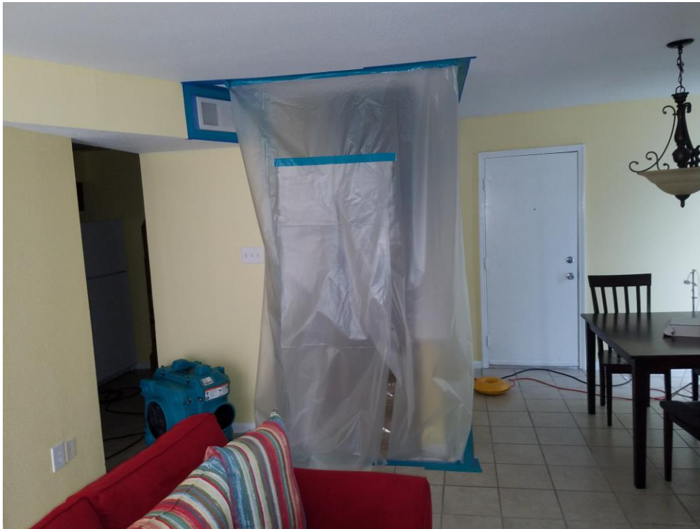
Entrance to stairwell containment, framing and sheetrock in utility closet
