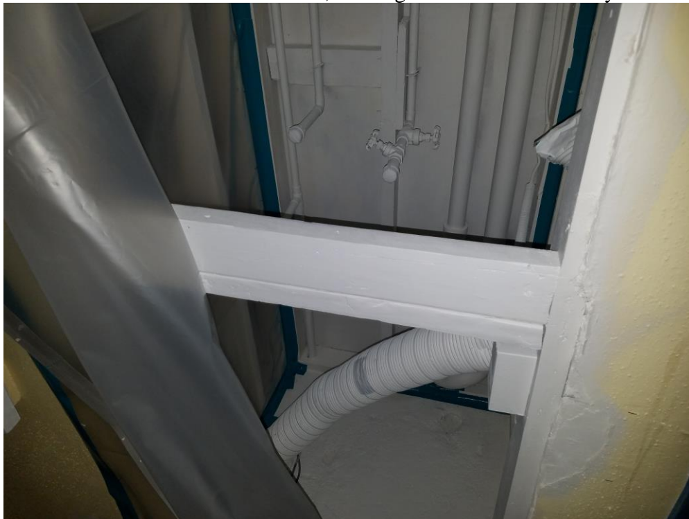
Entrance to stairwell containment, framing and sheetrock in utility closet
