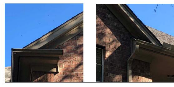
• Reset falling gutter with new gutter hangers and reconnect to downspout on front right side of home.
