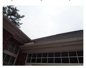
Gutters are needed at the front of the home, there is evidence of water penetration inside on the wood floors (see pictures under "F. Ceiling and Floors"). It may be advantageous to remove all the old gutters and install new 6 inches gutters which will divert a larger amount of water away from the exterior walls and doors.
