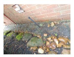
The gutter downspouts are terminating too close to the foundation; splash blocks are needed under the downspouts or downspout extensions are needed. Water runoff from the roof should be discharged at least 5 feet away from the home.
