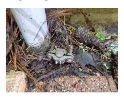
Note: The ground wire is not connected to the grounding rod with an acorn clamp. While this may not have been a code requirement when the home was built it is now a requirement for all TREC Licensed inspectors to call this item to the buyers attention.
