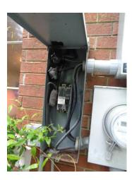
There were "white wires" attached to breakers. White wires are deemed neutral and must be identified as hot wires by tape or red or black paint at breaker end.
