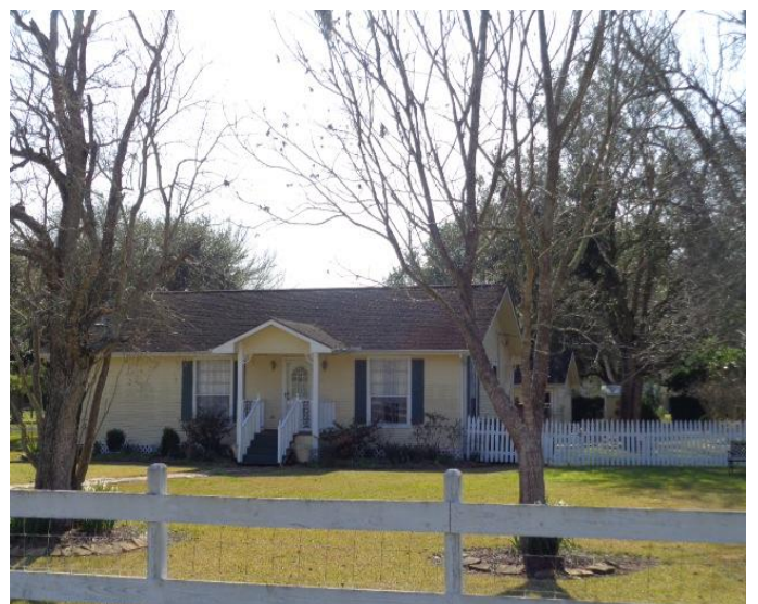
Street view of front from Lea Lane
