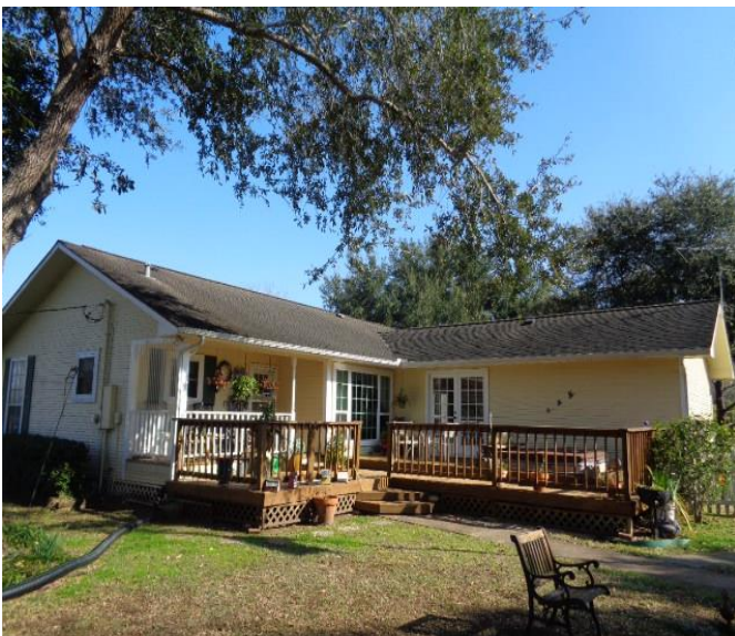
Back deck w/hot tub; French doors into master
