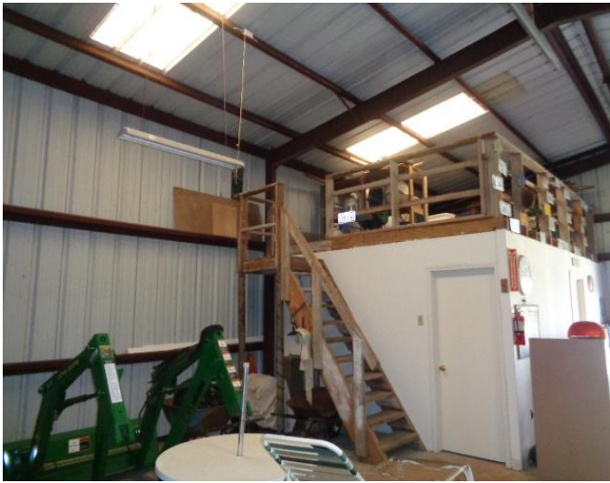
Stairs to storage area above office
