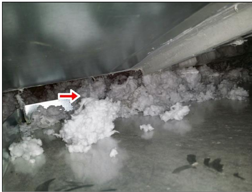
Insulation to be removed from pans
