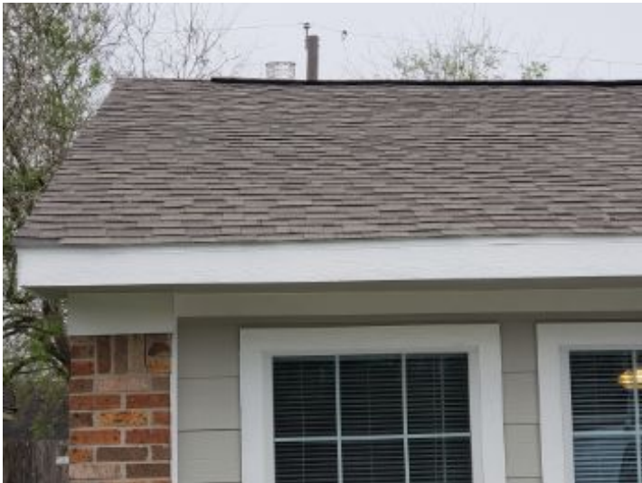
Roof shingles are 30 year warranted fiberglas laminated shingles, and in excellent condition.
