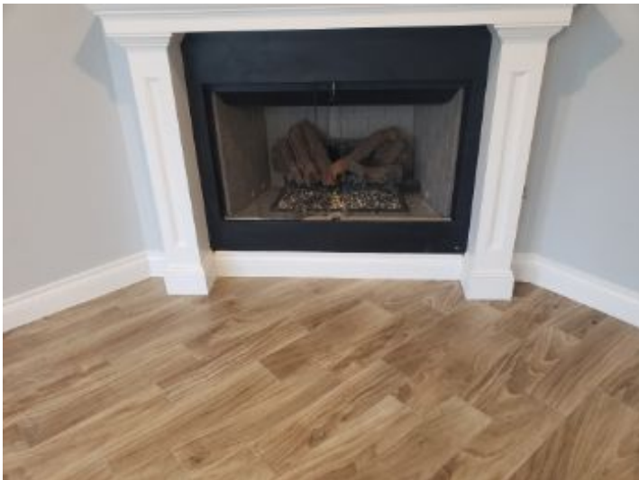
I could not get the fireplace to light and didn't detect gas coming out of the lighter when the valve was on. A remote control was not available and the switch to the right of the fireplace didn't do anything.
