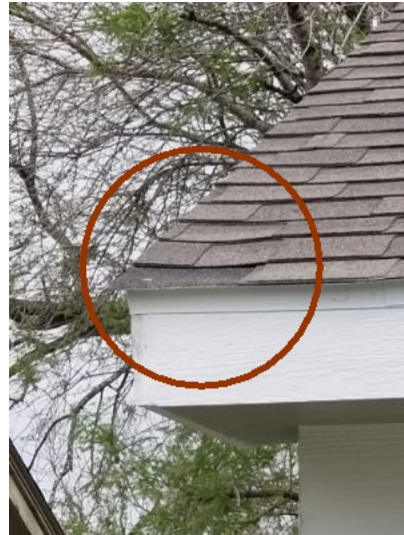
Front left corner of roof (over previous garage) missing shingles and needs repair.
