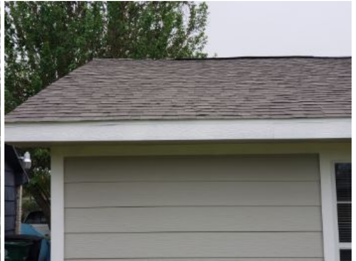
Front left corner of roof (over previous garage) missing shingles and needs repair.
