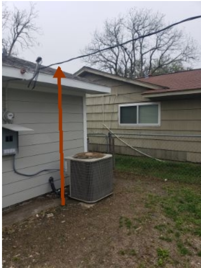
Electrical service wires and weather head installed too low for current requirements. They are at 8' from the ground and should be a minimum of 10' from the ground.
