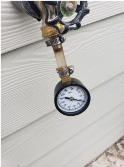
The anti static water pressure was observed at 60 PSI.
