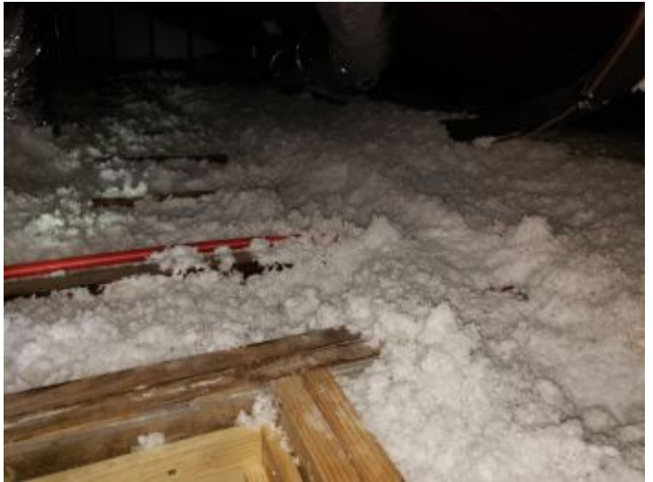
The loose fill attic insulation averages a depth of approximately 12".
