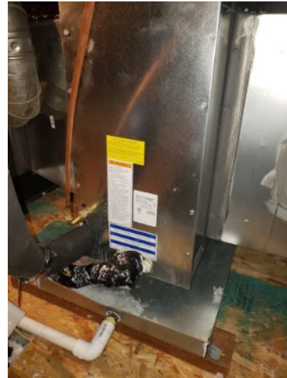
Brand/model: The condenser is a Payne model PA13NA048-C/serial number 1210X76136 13 SEER 4 ton unit manufactured in March of 2010 and the evaporator coil a Goodman Manufacturing model CSCF4160N6DA/serial number 1712000504 manufactured in December of 2017. Type of system: Conventional split system using R-410A freon to cool. Evaporator coil with drain pan and main/secondary drain lines.
