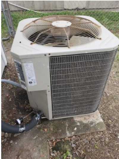
Brand/model: The condenser is a Payne model PA13NA048-C/serial number 1210X76136 13 SEER 4 ton unit manufactured in March of 2010 and the evaporator coil a Goodman Manufacturing model CSCF4160N6DA/serial number 1712000504 manufactured in December of 2017. Type of system: Conventional split system using R-410A freon to cool. Evaporator coil with drain pan and main/secondary drain lines.
