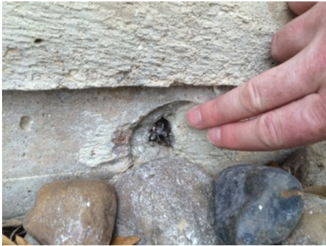
Rear: Exposed tendon head
