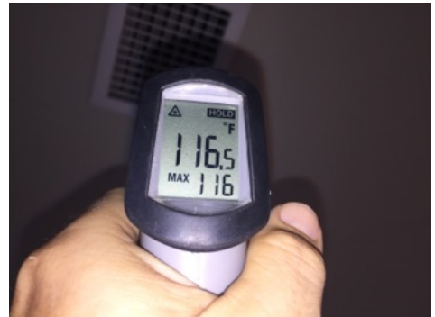
1st floor hot air temperature
