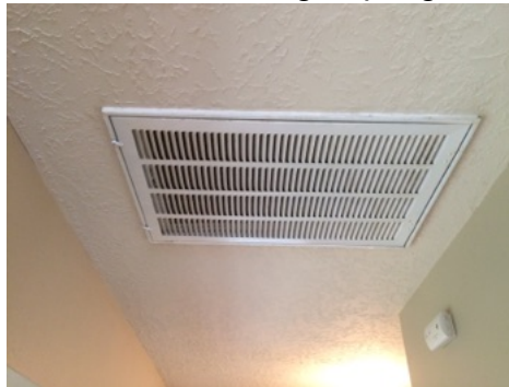
2nd floor dirty air filter size 16x25
