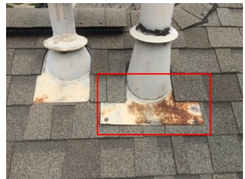
Corroded flashing
