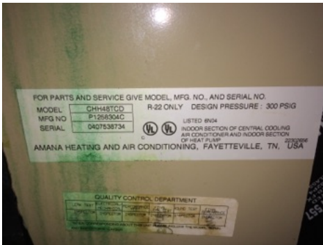
Evaporator unit 1 model and serial numbers
