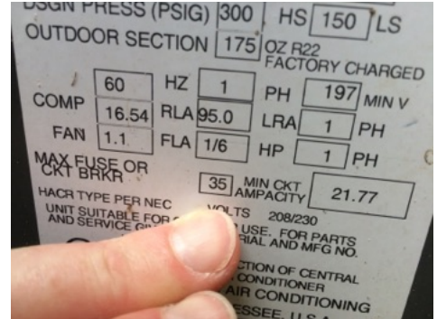
Condenser 1 max rated breaker 35 amps
