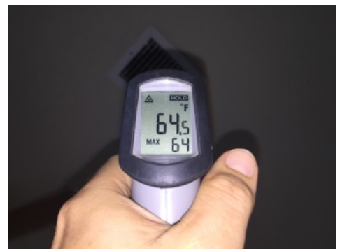
2nd floor: vent temperature
