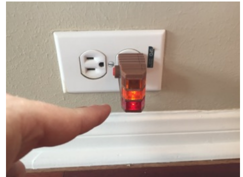
Dining room: reverse polarity at outlet under window
