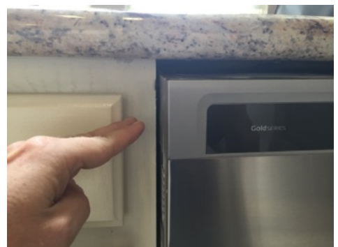
Door rubbed on left side
