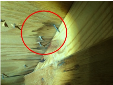
Moisture stain confirmed dry
