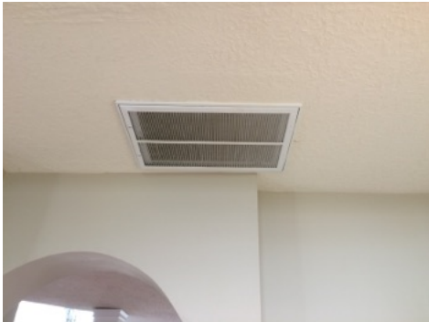
1st floor air filter size 16x25
