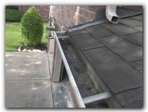
Evidence of improper sloping of the gutter was found as evident by a standing water in sections of the gutters. This problem can lead to future leaks.
