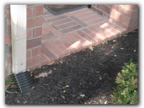
Loose gutter downspouts should be secured to insure proper function and prevent damage.
