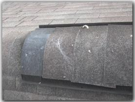
Evidence of loss of aggregate and exposed fibers were noted during the inspection of the roof covering as evident of aging.
