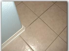
Loose flooring was noted on the second floor as evident by noise when walking. Recommend securing / re-nailing all loose flooring.
