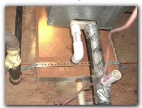
Air leakage was found at the evaporator coil housing of unit #2. Repair by a licensed HVAC contractor is recommended.
