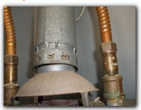
Noise was heard from the water heater during operation due to mineral deposits within the tank. A licensed plumber should be consulted to determine possible solutions for this problem. Replacement of the tank could become necessary to eliminate this problem.
