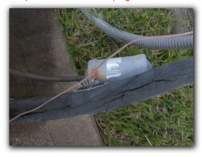
Damaged and missing insulation on the visible portions of the refrigerant lines should be repaired/replaced at unit #1.
