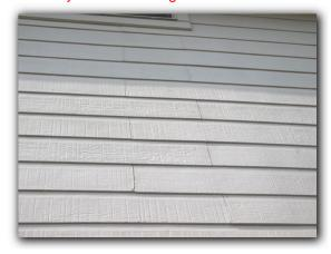
All exterior wall penetrations (electrical panels, electrical disconnects, light fixtures, etc. ) and openings (expansion joints, windows, door thresholds, etc. ) should be sealed with an approved material to prevent water penetrations into the wall cavities. Properly sealed exterior veneers help provide a barrier against the weather, insects, and enable environmental control of the interior spaces.
