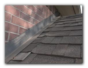
Damaged and / or missing shingles were found during the inspection of the roof covering. Recommend repairs by a qualified tradesman.
