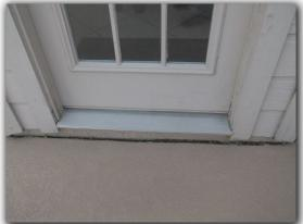
Damaged and missing sealant / caulking was found at joints, transitions, and voids on the exterior veneers. This material acts as a moisture barrier to prevent water from moving to the underlying wall cavity. The re-sealing of the exterior veneers should be considered.
