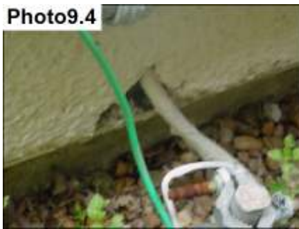
Seal all penetrations
