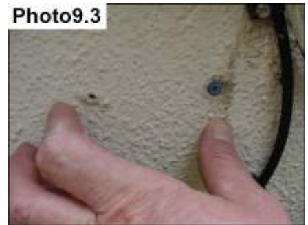
Seal all fasteners
