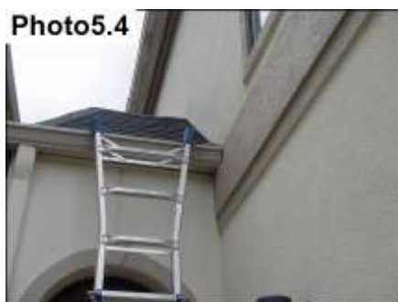
Kickout flashings are present and sealed
