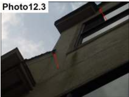
Seal all flashing terminations
