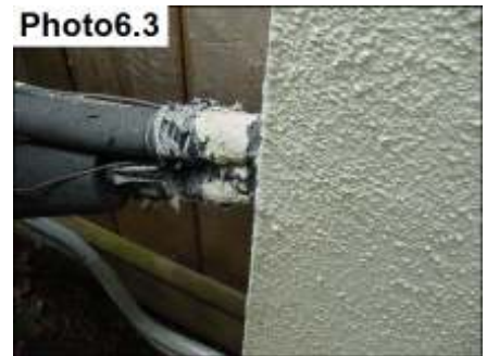
Seal all penetrations as needed
