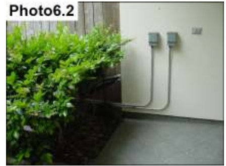
Seal all penetrations as needed
