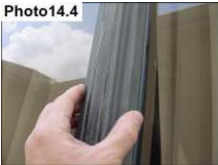
Seal all mullions on windows / Wet glaze all fixed windows
