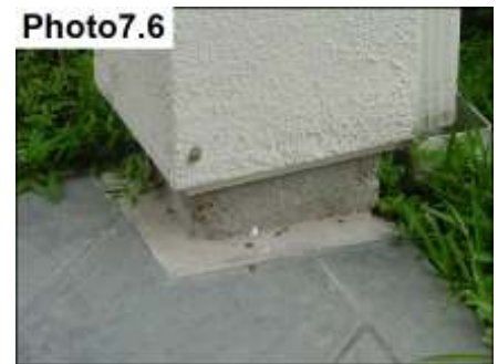
Column base is on a concrete footing
