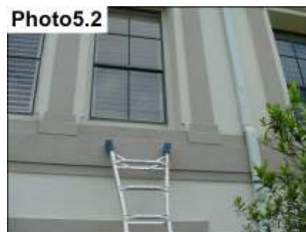
Some sealant separation noted
