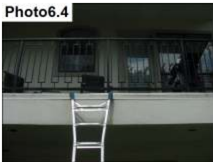
Seal all railing bolts / fasteners
