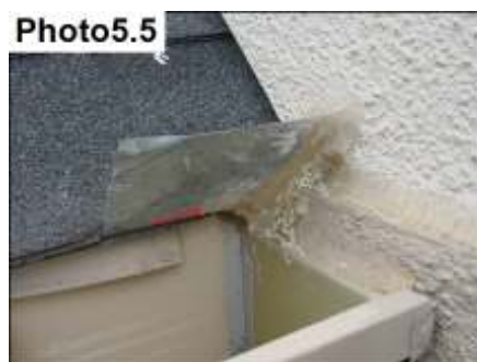
Kickout flashings are present and sealed
