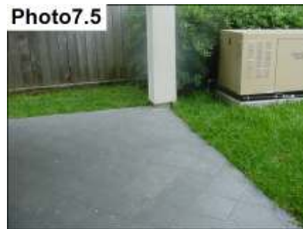
Column base is on a concrete footing
