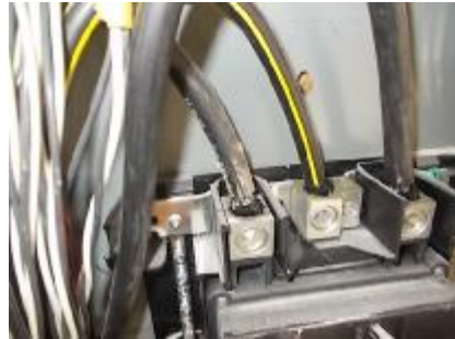
Electrical panel/main service conductors/main
