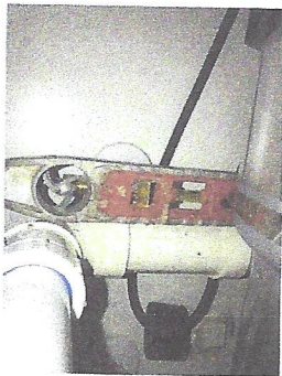
30. Missing escutcheon has been replaced (see picture) and it is draining properly.
