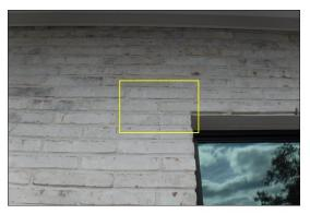
Rust staining observed on walls below penetrations (front iron lanterns and doorbell)
