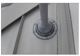
Daylight observed in attic around water heater exhaust vent penetration. This could be a potential point of water penetration.
