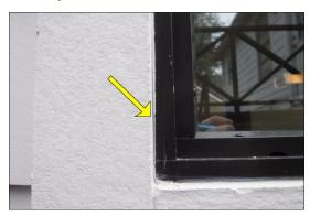
Staining observed on side of guard east side of front guard wall, possibly due to lack of sunlight.
