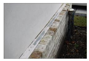
The guard wall at front of house at southeast corner is pulling away from structure. Large gap observed between wall and house that may allow water accumulation.
