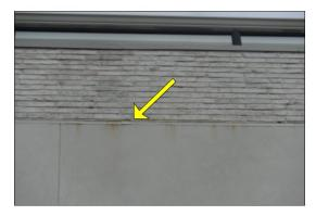
Possible water entry from joints and/or penetrations in stucco siding, Recommend sealing / caulking around all cracks and exterior siding penetrations including but not limited to light fixtures, electrical outlets/service panels, dryer, bath vents, etc.
