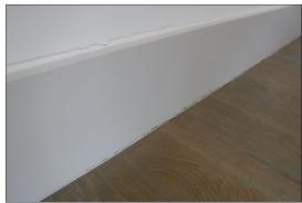
Some separation observed between wood planks at multiple locations; third floor near balcony door and first floor near kitchen.
