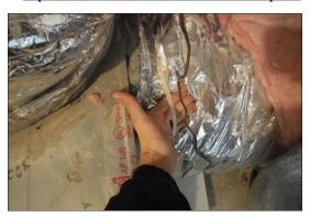
Some flex duct observed to be improperly routed with sharp bends and / or excess material in bends. Improper routing increases frictional loss in the duct and reduces heating and cooling efficiency. Radius at centerline of the bend should be no less than the diameter of the duct.
