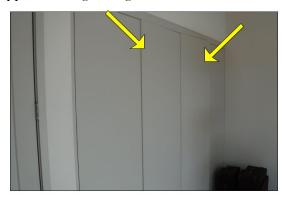
Cosmetic cracks and/or repaired cracks in sheetrock observed over some / many doors, windows, and/or corners.
