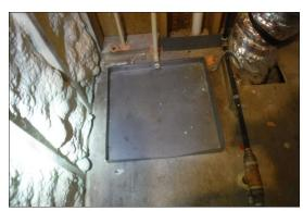
The condensate drain line and components do not appear to have been installed properly to allow for proper drainage. Hose is missing required drip loop and the line is crimped at one or more locations and not properly secured in drain. Recommend further evaluation by a qualified professional.
