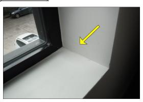
Water penetration observed at the following location(s): at third floor fixed window. Recommend further evaluation/repair.
