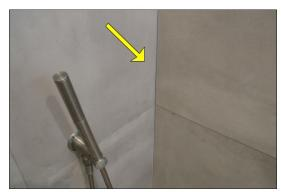
Observed level or improper sloping of shower window sill tile, sill should slope towards interior of shower not back towards window frame.
