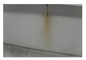
Head flashing missing over some windows / doors. Head flashing helps prevent water penetration. Without head flashing windows/ sealing must be maintained as the only defense against water penetration.
