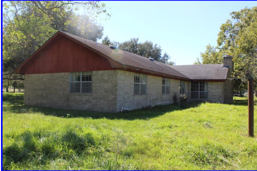
Exterior view of Residence from the east
