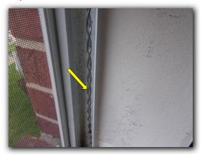
\* There are various windows in the home that have previous water damage at the window sills – these sills were dry at the time of the inspection but need to repair any damage and monitor.
