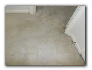
\* The flooring in the upstairs of the home has some sloping – this sloping is fairly common from settlement but need to monitor as this may be a sign of movement in the framing.
