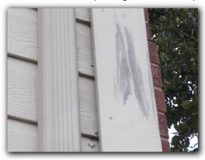
\* There is various damage and deteriorated areas in the exterior siding and trim of the home such as on the rear of the home — need to repair the damage to the siding and trim of the home and seal with caulking and paint.
