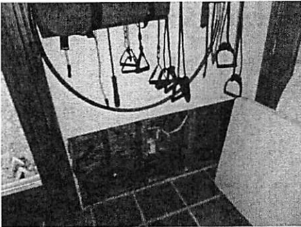
Pool room door frame
