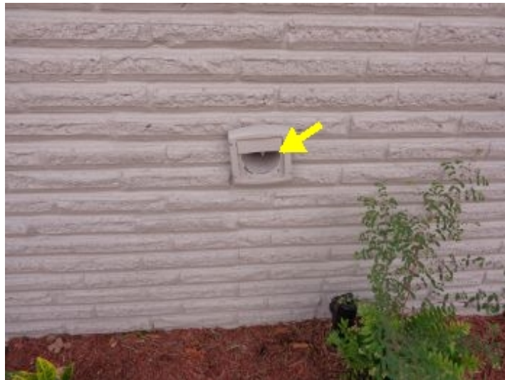
Exterior dryer vent cover - is damaged
