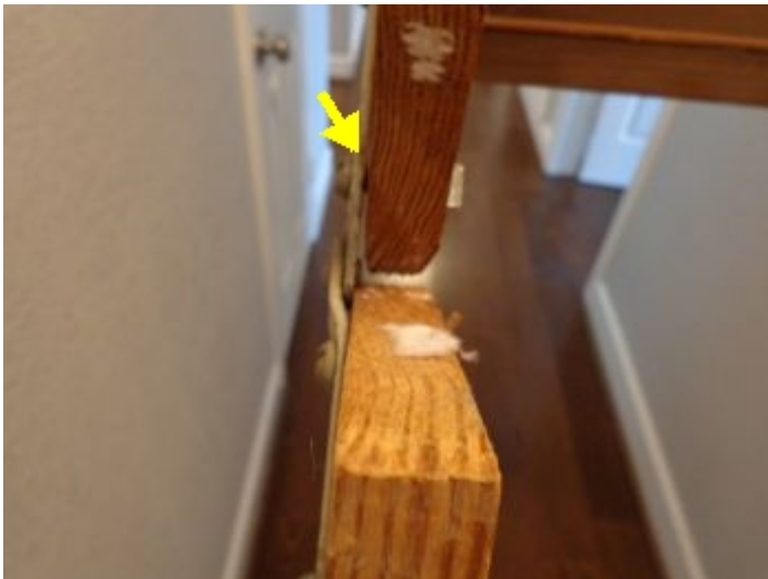
Attic access ladder - Hardware is loose, damaged or missing. - Recommend repair before using for safety. Periodically inspection of the metal brackets and hardware is needed as they tend to loosen. Tighten as needed.
