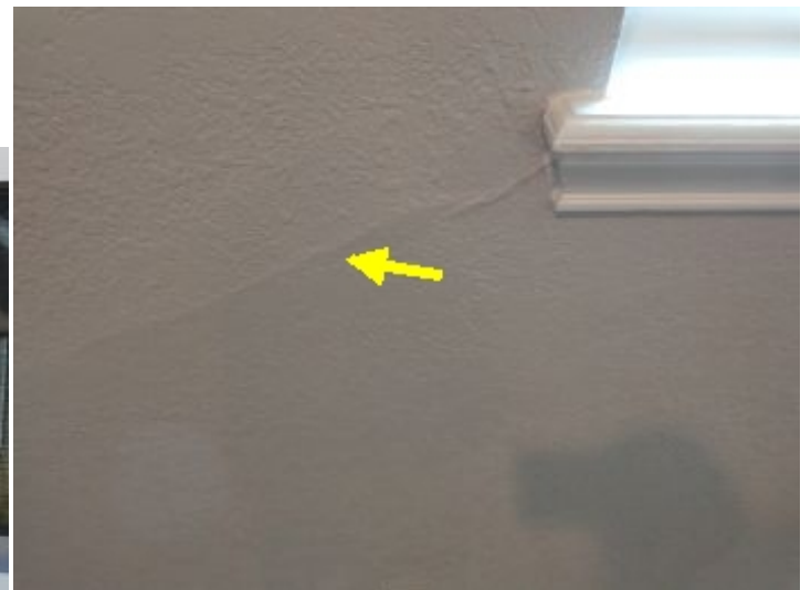
Note: Observe previous sheet rock crack has been patched and repaired and painted Master bedroom left wall
