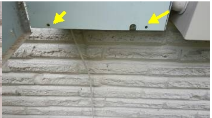
Screws missing for dead front cover plate – Note: Screws should have a flat tip, not pointed
