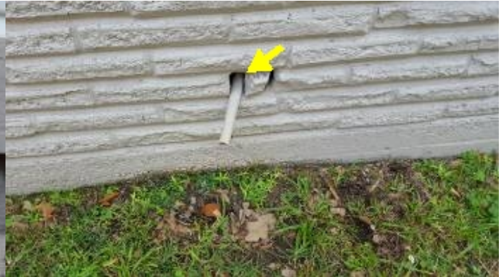
Hole in exterior wall with drain line running thru it is not caulked and sealed - left side of the house.
