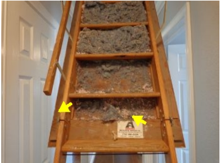
Attic access ladder - Insulation displaced on door - I recommend replacing with Foam board type material sometimes works better as it will not slide down or move when ladder is being used etc. Also adding weather stripping around the edge - To improve energy efficiency.
