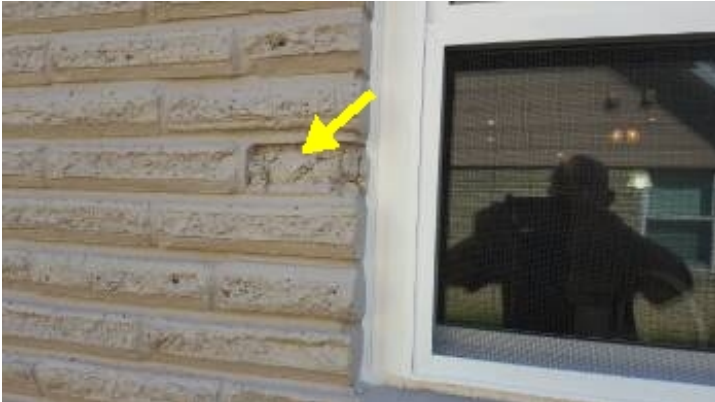
observe damage brick right side of house next to the kitchen window
