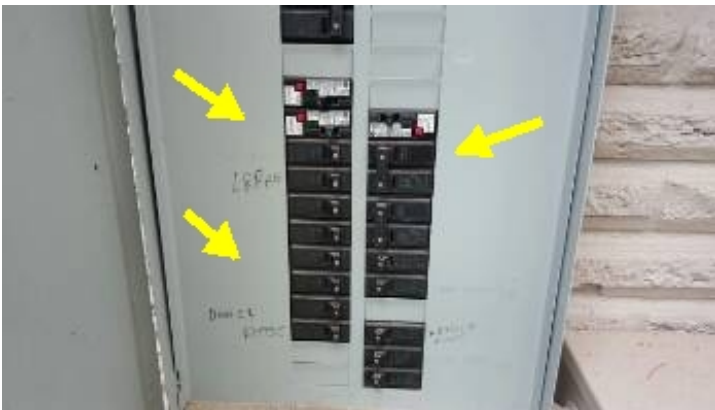
Label all circuit breakers - Panel board circuit breakers are not completely labeled, or the labeling has faded. – Recommend clearly labeling all circuit breakers.
