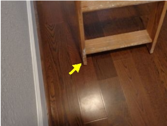
Attic access ladder - It is recommended that pads be installed at the base of the stairway unit "legs", to prevent wood flooring damage.
