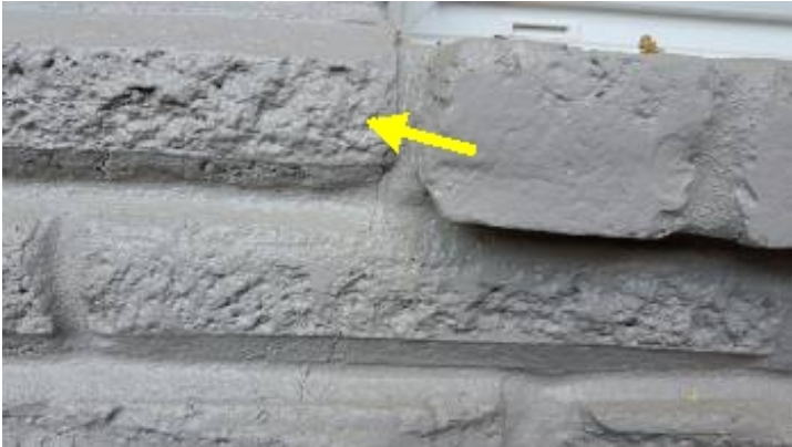
observe damage brick right side of house next to the kitchen window
