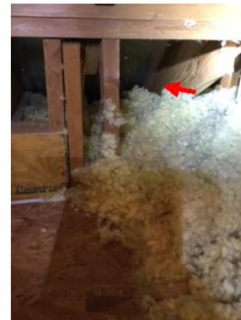
Blocking soffit vent
