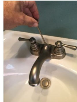
Linkage broken
