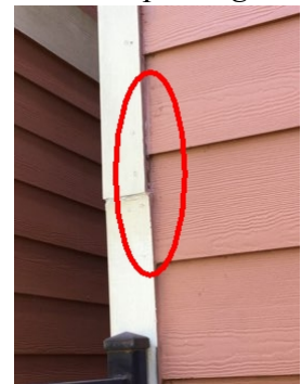
Sealant deteriorating
