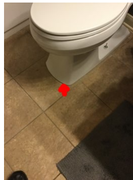
Missing sealant
