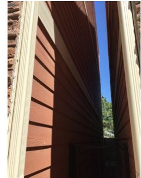
Unable to inspect
