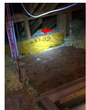
Blocking soffit vent
