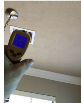
2nd floor supply vent 57%.
