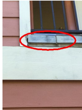
Sealant deteriorating
