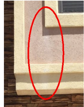
White efflorescence
