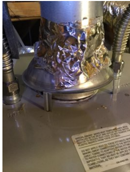
Improper connection
