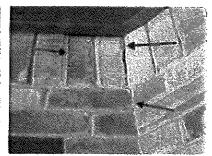
Mortar repairs were observed in the brick veneer at the rear patio and right side exterior walls.
