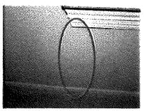
Water staining was observed on the wall near the front door. This area was dry at time of inspection.
