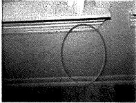
Minor cracking and separations of the drywall tape joints were observed at the kitchen near the front entrance.
