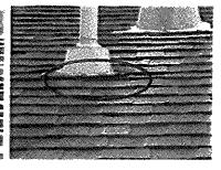
A satellite dish is mounted to the roof covering. Higher than normal maintenance should be expected in this location.
