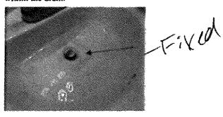
• The drain stoppers did not seal and hold water at the left side guest bathroom sink and master bathroom right sink.
