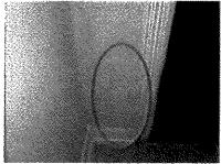
Water staining was observed underneath the living room rear window. This area was dry at time of inspection.
