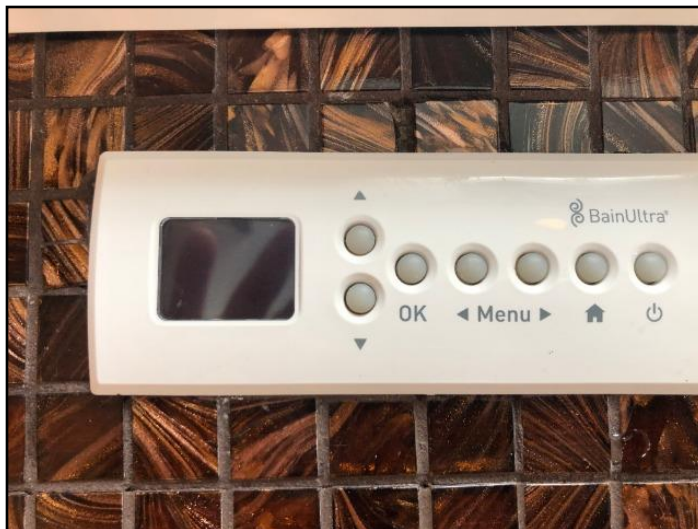
Control for whirlpool is not functioning
