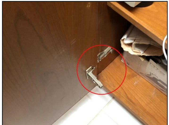
Pieces missing or loose
