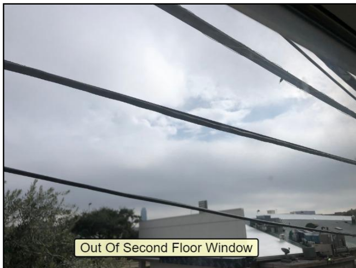
Inadequate window or door clearance
