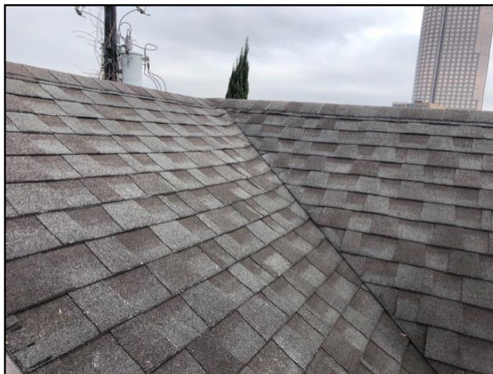
General view of Roof
