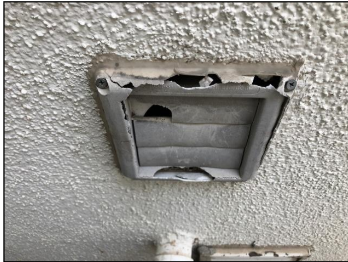
Cover damaged
