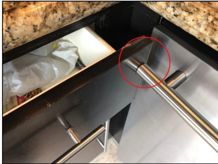
Drawer does not fully open.
