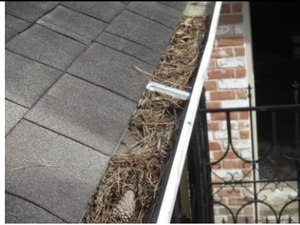
Pine needles in gutter
