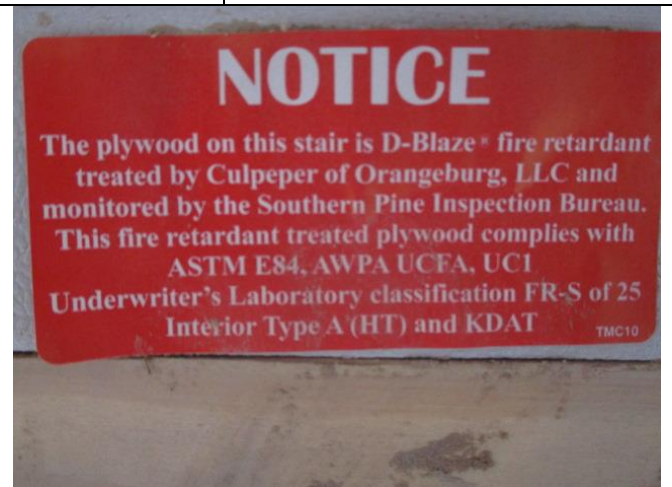
Sample label to indicate cover is fire-rated
