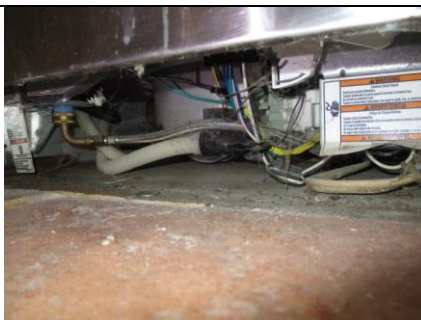
Dishwasher kick plate was removed to inspect for water leakage
