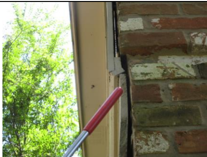
No sealant. Bees entering wall cavity at this balcony location.
