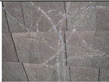
Shingle damage
