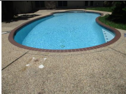
Separate fence is not installed around pool-spa
