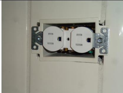
Example of extension ring installation
