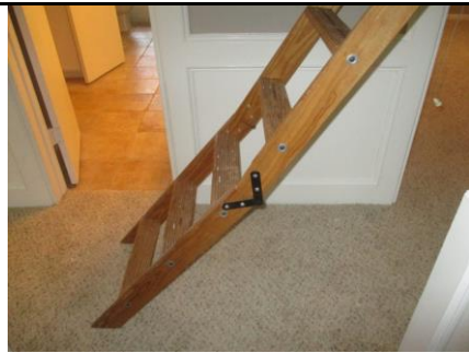
Stairway opens incorrectly
