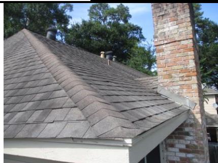
Roof surface was walked-Bird's eye view
