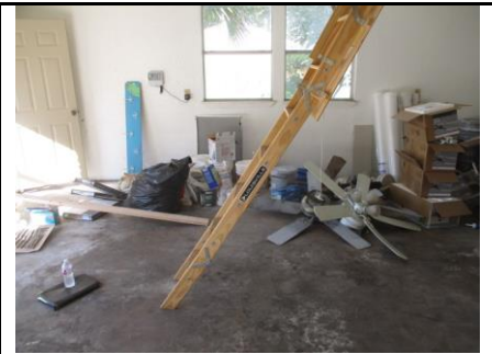
Stairway opens incorrectly
