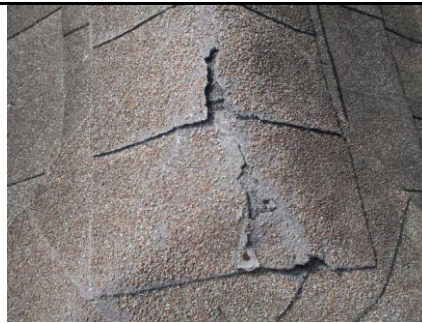
Shingle damage
