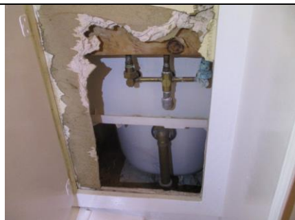
Bathtub access covers were opened-removed to inspect for water leakage.
