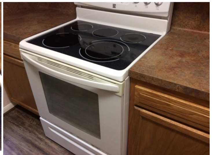
Anti-tip device not installed on the freestanding stove
