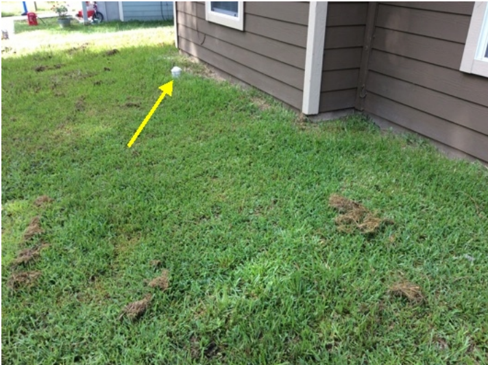
Main sewer clean out is in front of the house
