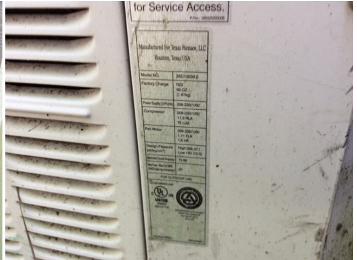
Nameplate information Texas Furnace, 2.5 ton
