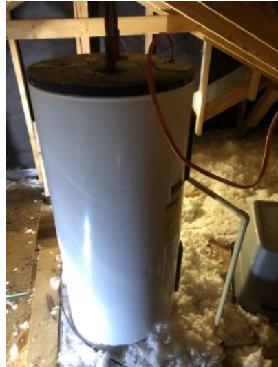
40 gallon, electric, water heater
