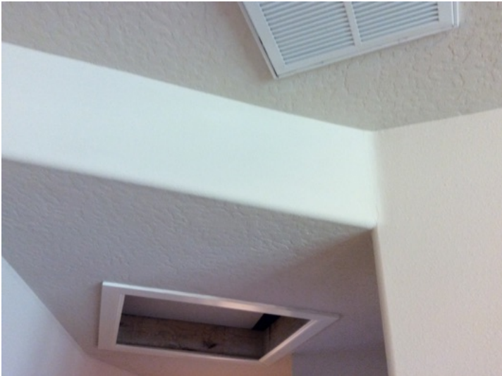
Furnace would not operate at the time of the inspection
