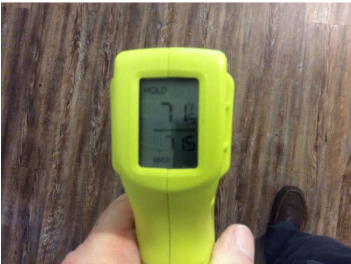
Cooling return temperature 71°
