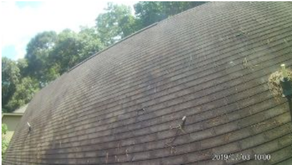
Various Angles and Views of the Roofing System
