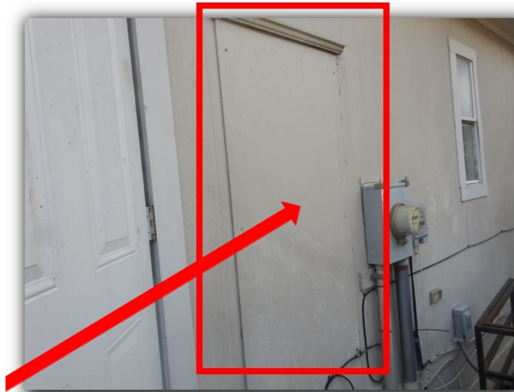
Water heater Temperature and Pressure Relief Valve
