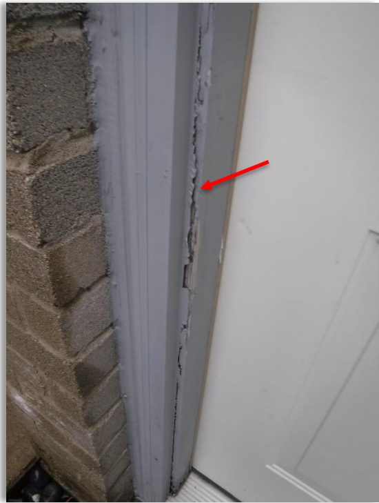
c. Sign of moisture damage and rot wood observed on the front door's jambs; recommend repair and re-paint;
