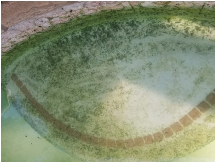
Pool surface appeared to be in need cleaning and repair and may possible need resurfacing. We recommend consulting with a pool resurfacing contractor for further evaluation.
