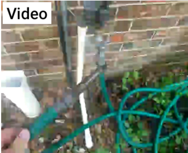
Water was running continuously at back yard exterior spigot. Shut off valve may be in need of repair.
