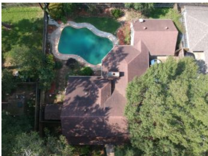
Structural Systems Roof Covering Materials
