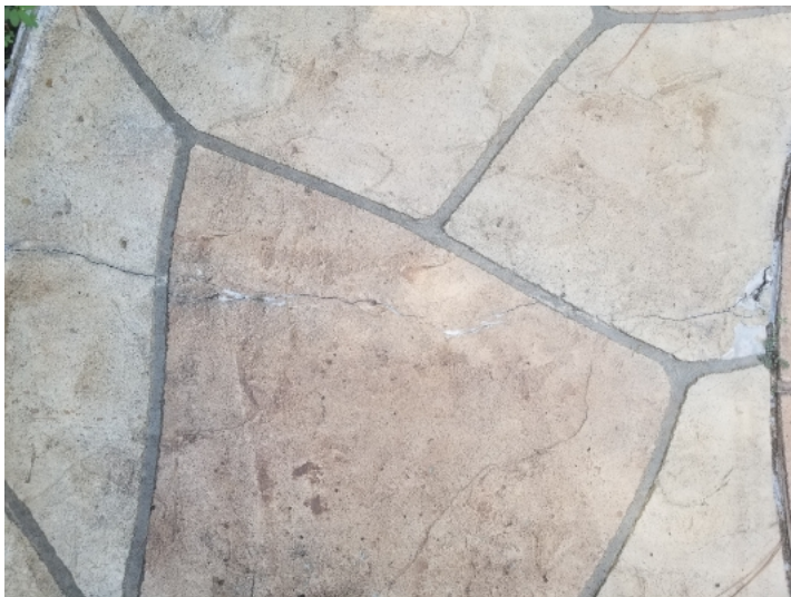
Decking appeared to be in okay condition. Some cracks were observed.
