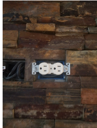
Outlet cover was missing in the living room at the fireplace.
