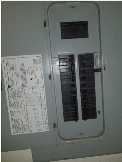
All breakers for the panel boxes and/or sub panels must be clearly and permanently labeled for identification of particular circuit.
