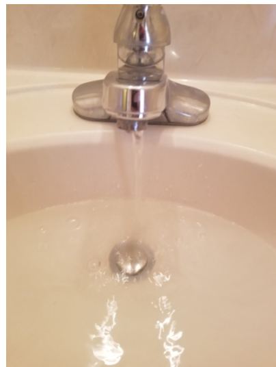
Low water flow was observed at the kitchen sink and 2nd level guest bathroom sink.
