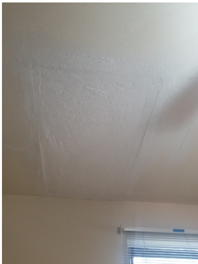
Full size attic entry was removed.
