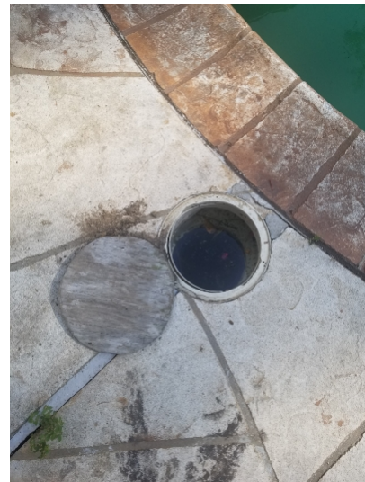
Skimmers were observed and appeared to be functioning as intended. 1 skimmer was missing the cover.
