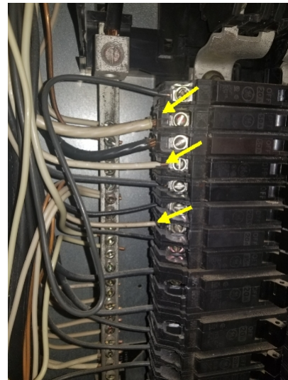
White wires were connected directly to breakers in the panel. Typically white wires should be designated as neutral only. These should be marked appropriately.
