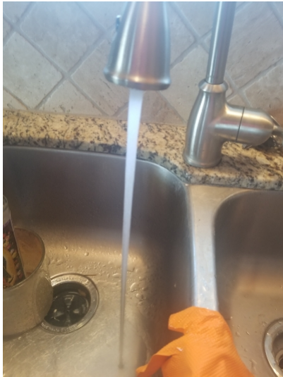
Low water flow was observed at the kitchen sink.
