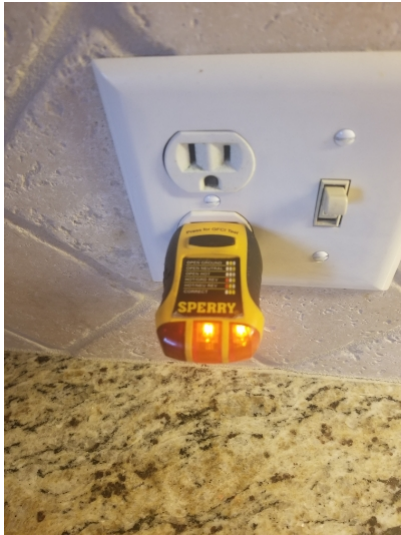
GFCI outlets were not present and functioning in the kitchen, bathrooms, garage and exterior.
