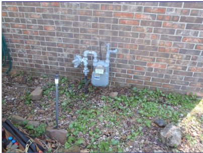
A. Item 1(Picture) Foundation below grade at back of home.
