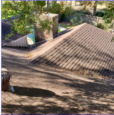
C. Item 6(Picture) General view.
