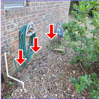
B. Item 1(Picture) Soil in contact with wall coverings at left side of home
