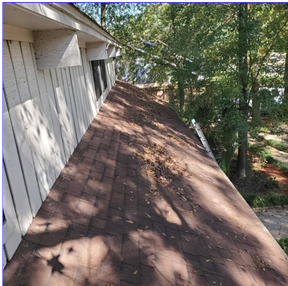
C. Item 1(Picture) General view.
