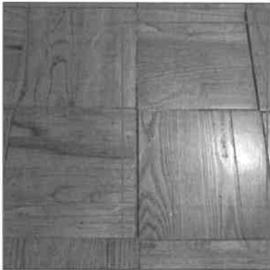
A. Item 21(Picture) front secondary bedroom
