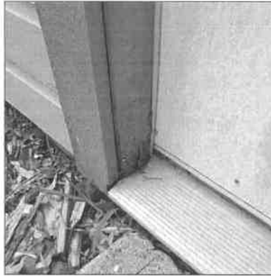
G. Item 1(Picture) right side of home
