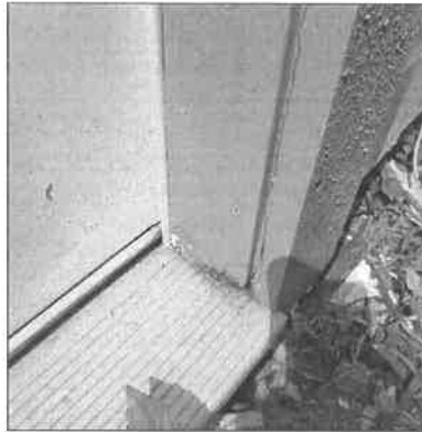
G. Item 2(Picture) right side of home
