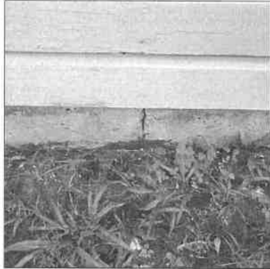
A. Item 1(Picture) right side of home
