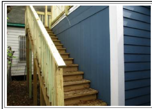
Stairs to upper deck
