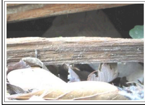
View of old beam under house
