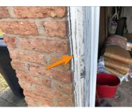
6: Exterior- Caulking: Missing Around Window Frames
