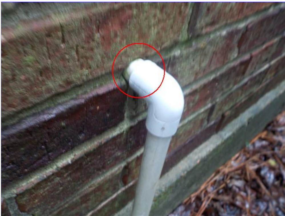
A. Item 2(Picture) PVC going in
