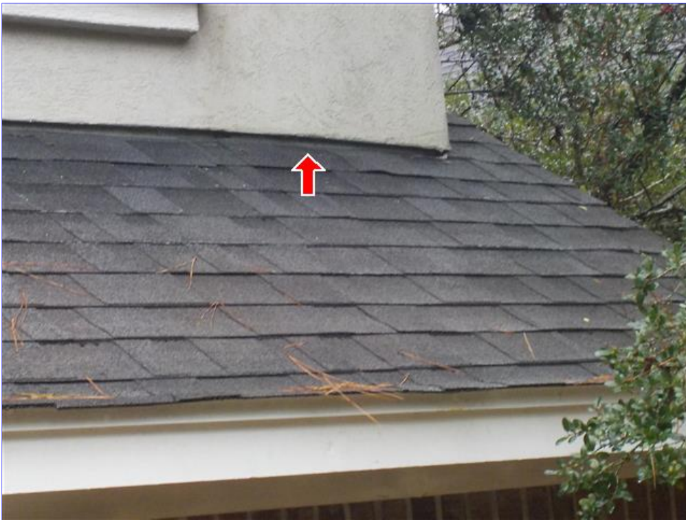
C. Item 2(Picture) Siding should have a 1in gap to the shingles
