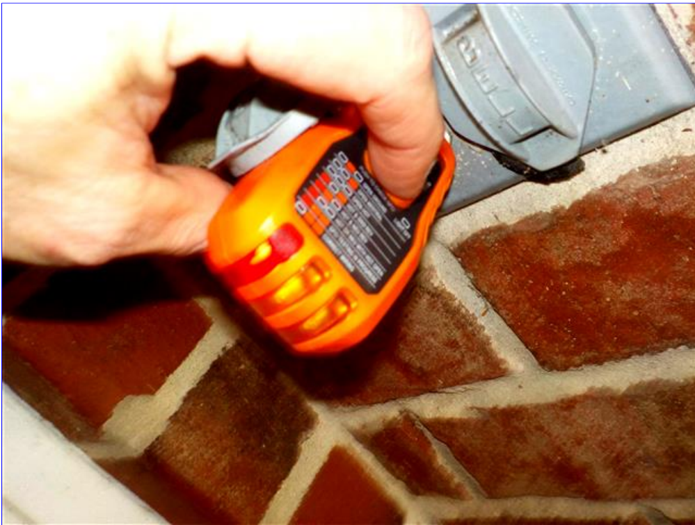
B. Item 4(Picture) Interior & exterior inspected
