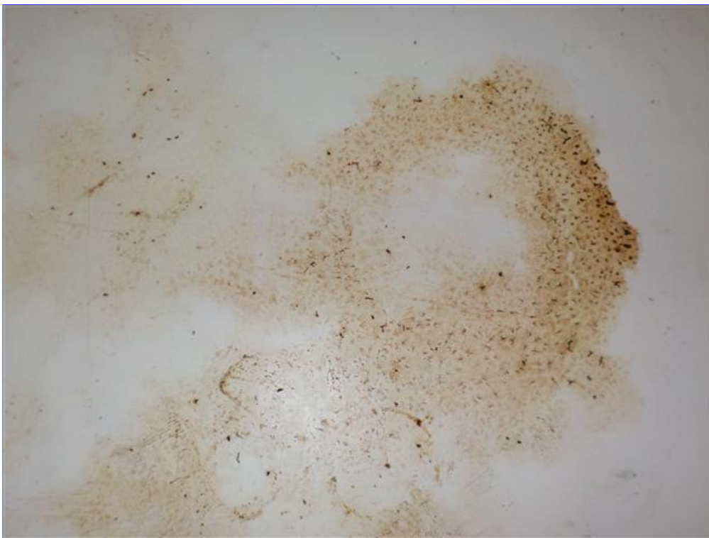
E. Item 2(Picture) Counter tops have stains
