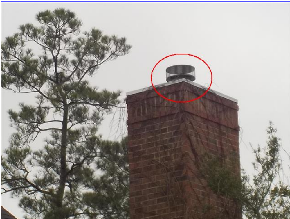
I. Item 2(Picture) Chimney vent cap
