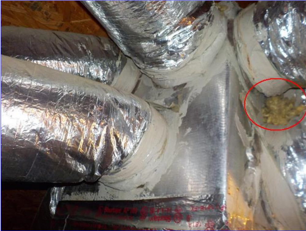
C. Item 9(Picture) Mastic should be properly applied
