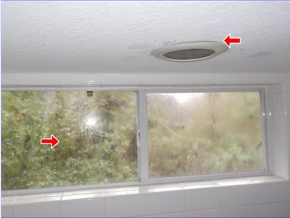
G. Item 5(Picture) High humidity evident by window condensation
