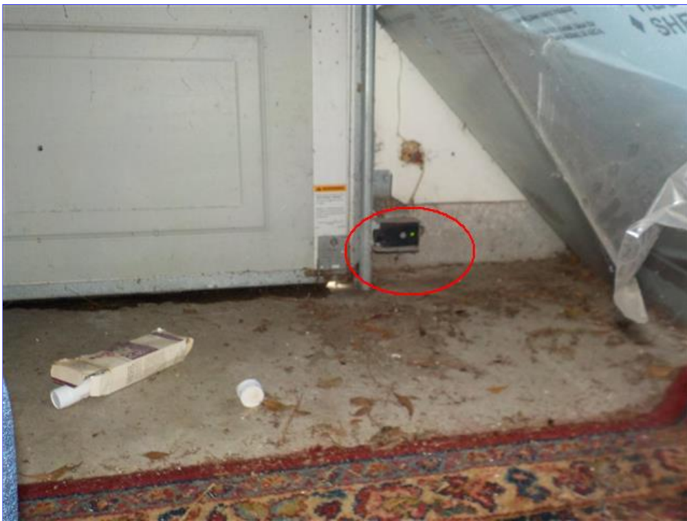
H. Item 2(Picture) Should be 6in from the center of the eye, its within tolerance
