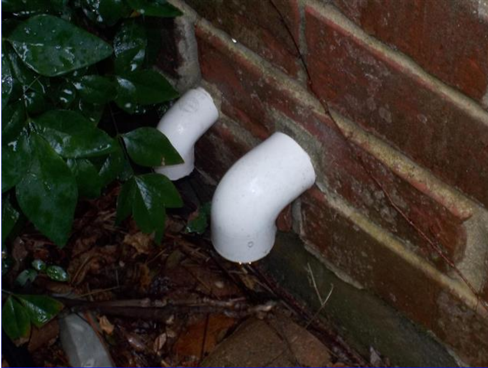
B. Item 1(Picture) Water heater drains add elbow
