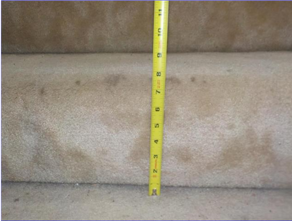
H. Item 1(Picture) Here we test if the stairs are within tolerance
