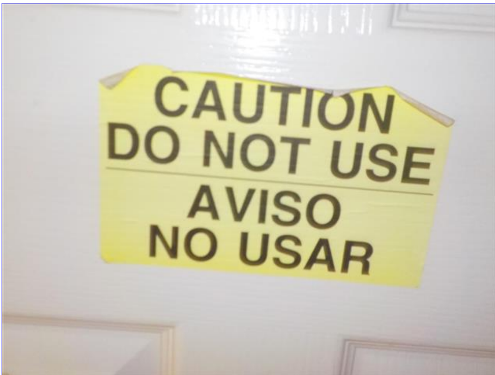
F. Item 2(Picture) Door stops not all in good condition
