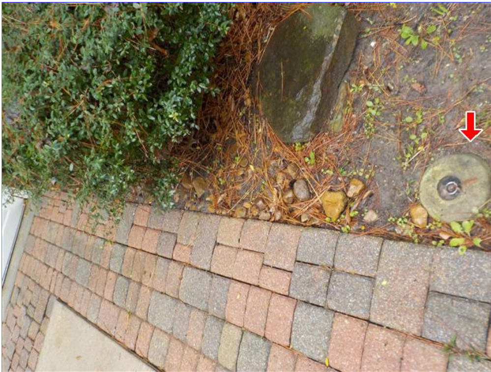
J. Item 2(Picture) Sprinkler will be hard to service
