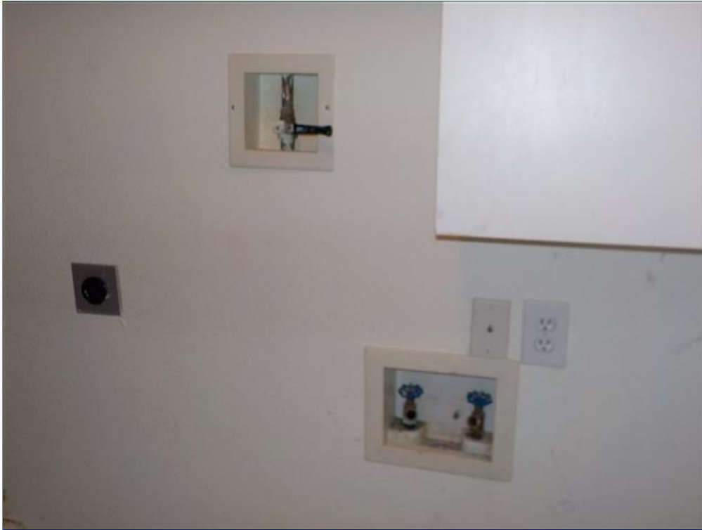
D. Item 23(Picture) Washer Dryer room
