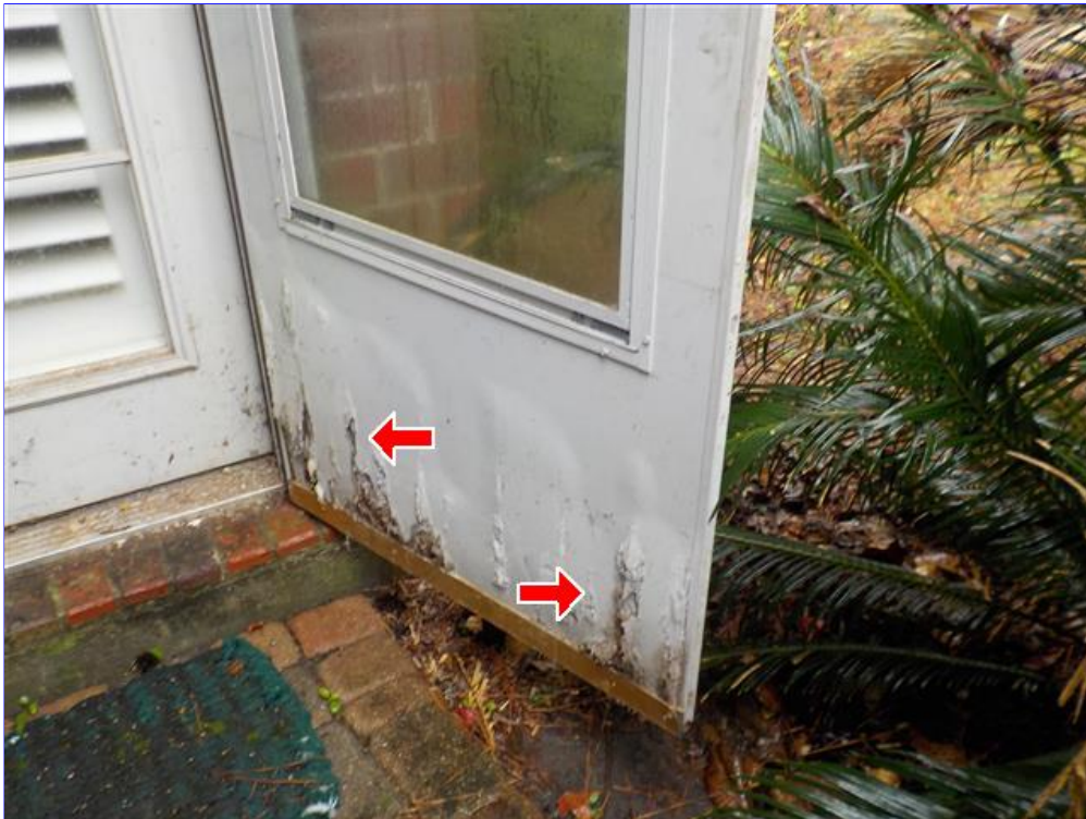
F. Item 3(Picture) Moisture damage possible wdi and wdo wood destroying insects and wood destroying organisms
