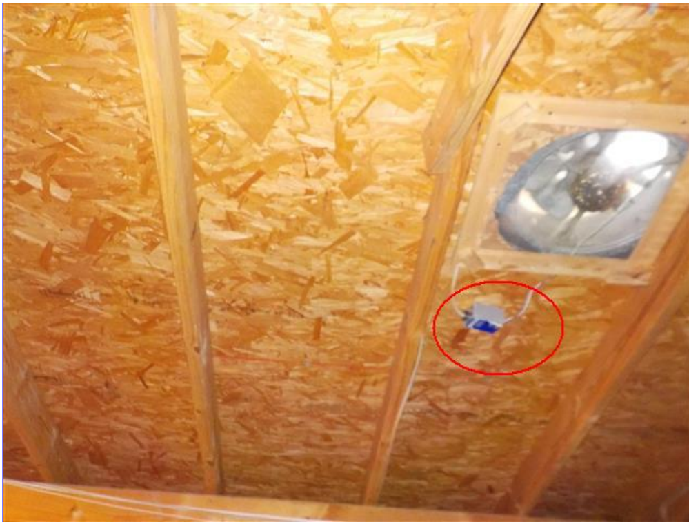
C. Item 12(Picture) Thermostat controlled vents
