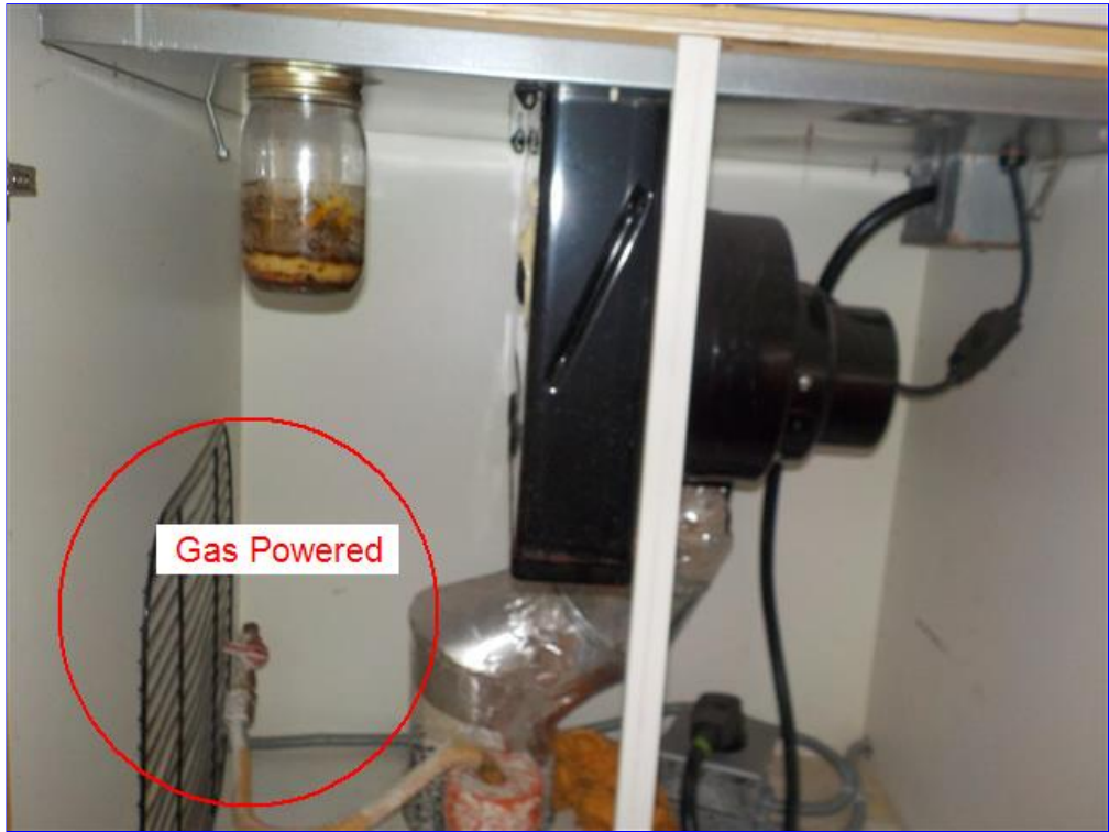
D. Item 3(Picture) Vents to kitchen
