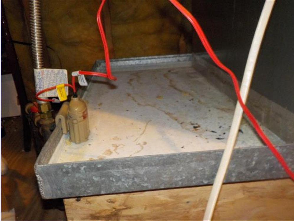
C. Item 11(Picture) debris in ac pan
