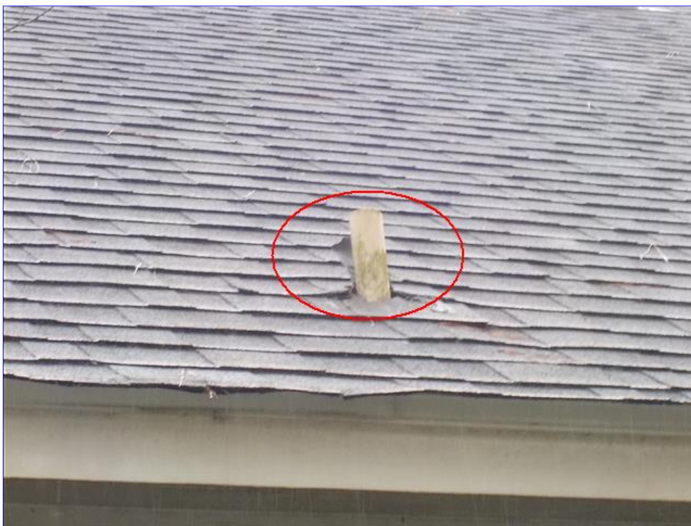
C. Item 2(Picture) Should be properly sheathed and PVC should not be used in this format
