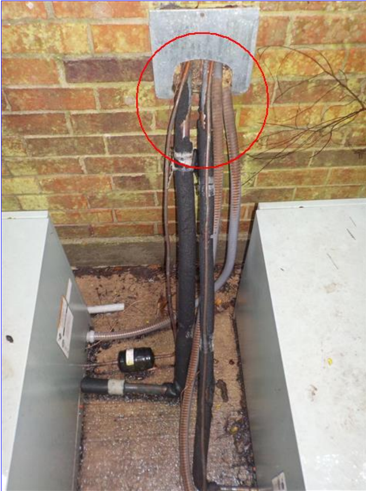
A. Item 3(Picture) Blocked well
