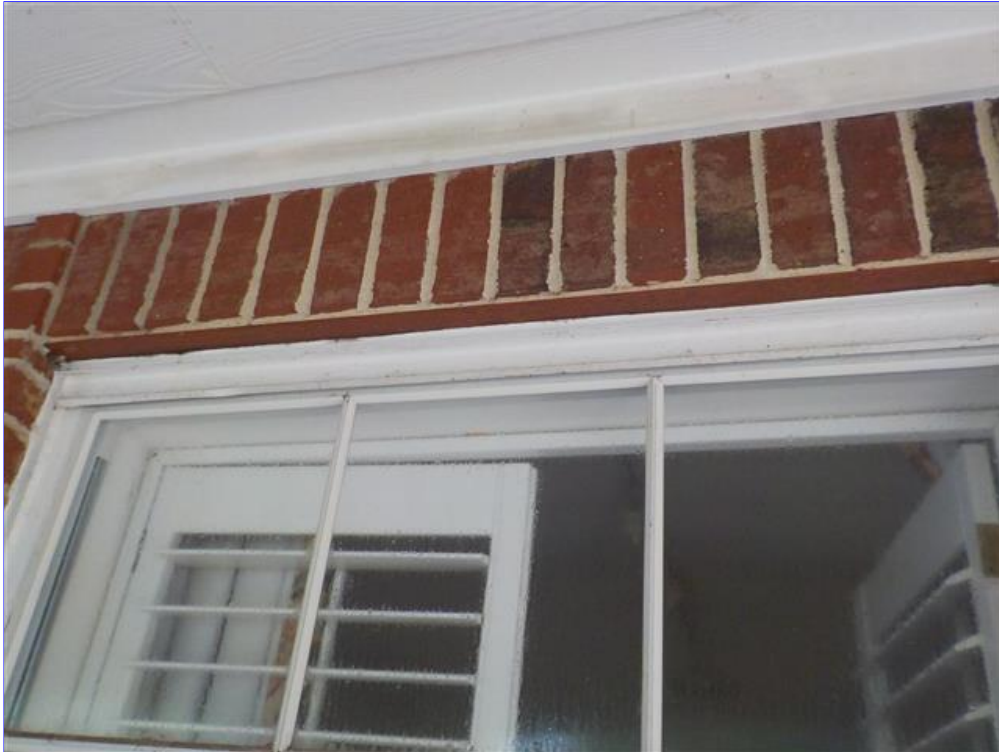
D. Item 16(Picture) Be sure lintels are in good condition
