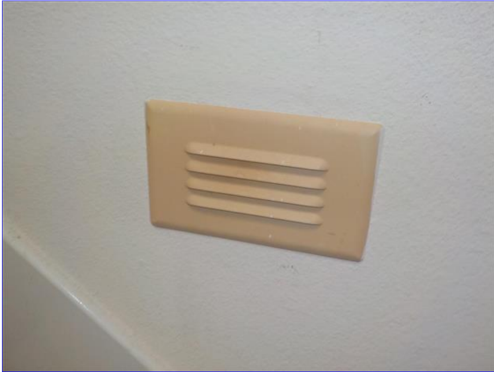
B. Item 11(Picture) Lights on the stairs
