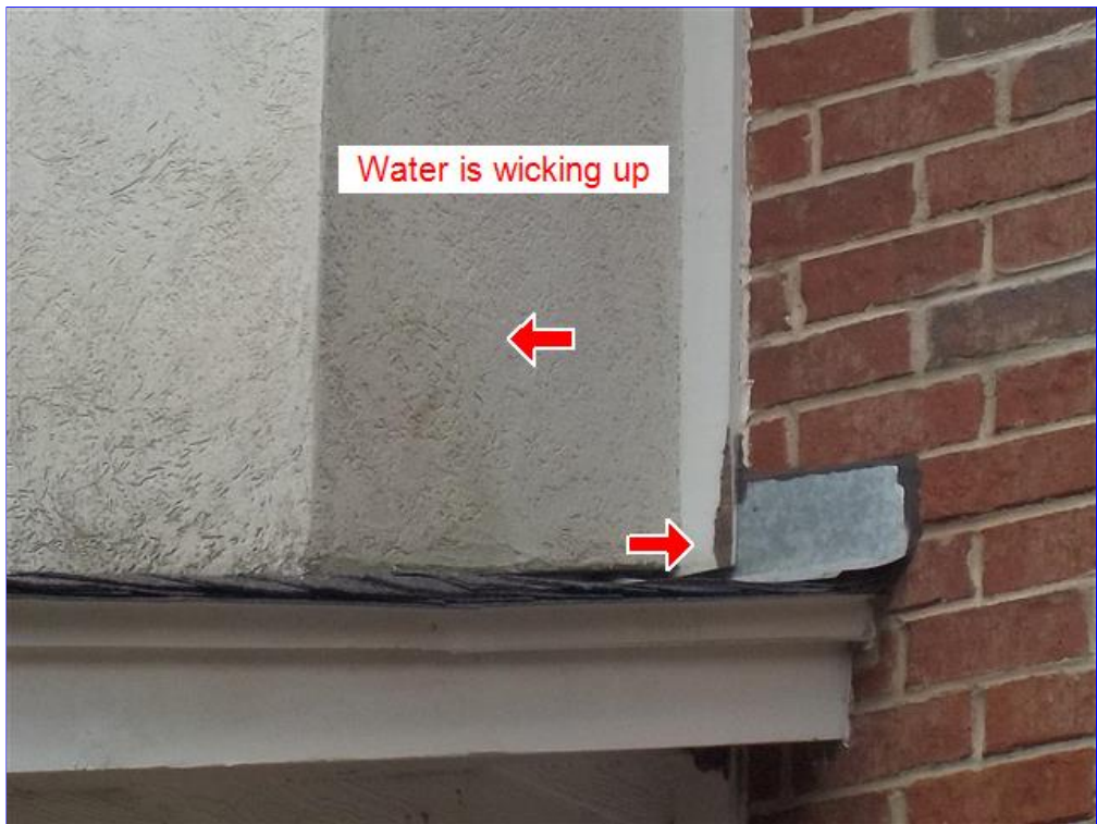
C. Item 3(Picture) Flashing needs to be followed through
