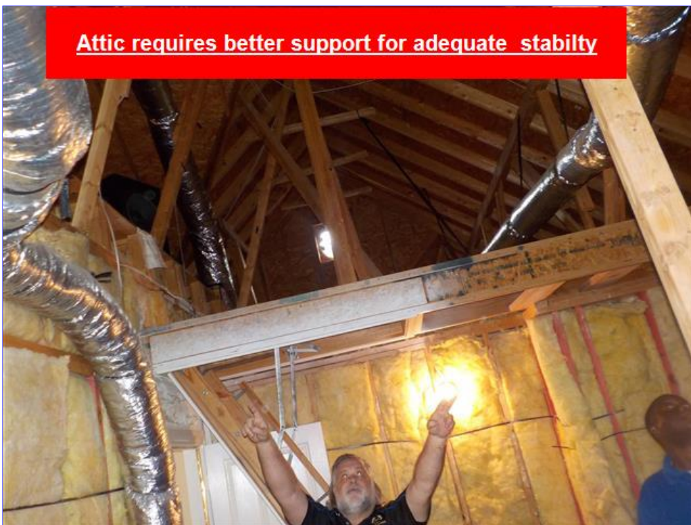
C. Item 26(Picture) Be sure the structure is fully supported.
