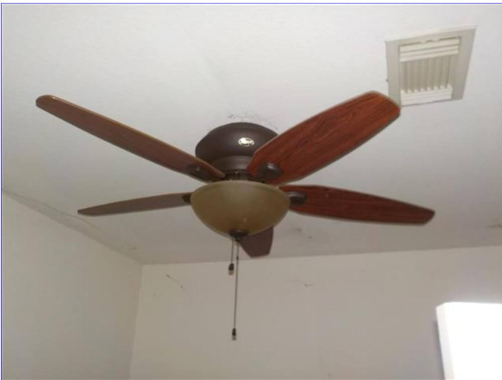
B. Item 10(Picture) Ceiling fan is in the garage
