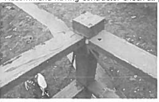
The above picture shows the wide space between the horizontal porch railings and does not comply with current standards.
