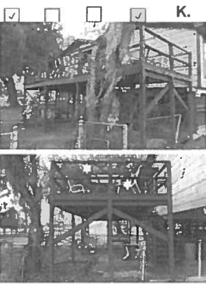
The above picture shows the wide space between the horizontal porch railings and does not comply with current standards.
