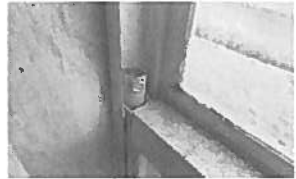
Spring balance have fallen on the back middle window in the living room.
