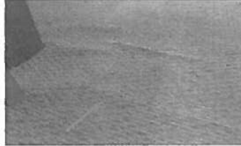
Ripples observed to the carpet in the master bdrm.
