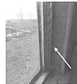
The spiral balance has fallen on the bdrm 2 right window.
