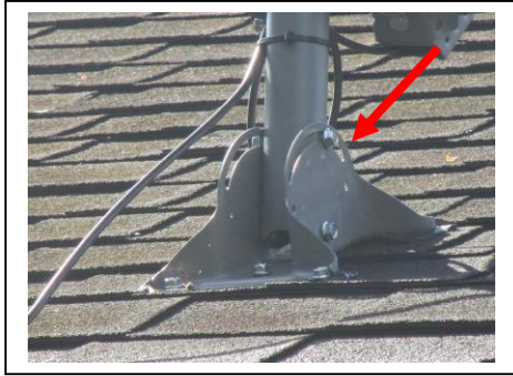
Satellite Dish Installed On Roof
