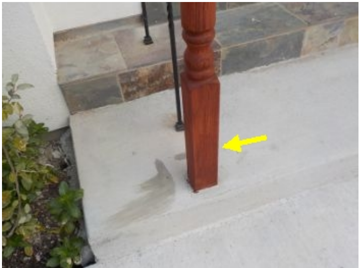
Handrail was loose at the front porch.
