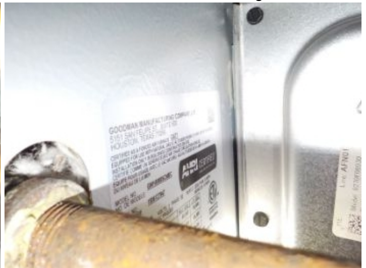
Furnace access door was missing a fastener.
