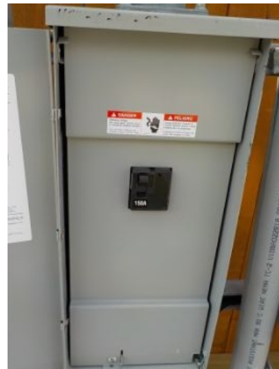
The dead front cover was not properly flushed with the panel enclosure. The panel enclosure appeared to be recessed well behind the drywall creating a gap between the enclosure and dead front cover.
