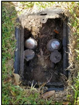
Front near sidewalk, water meter
