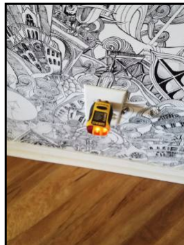
Living room, loose receptacle
