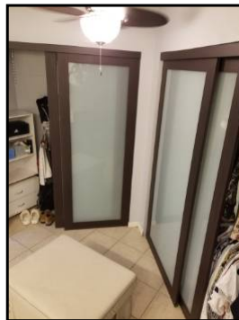
Master closet doors are missing bottom guides/tracks
