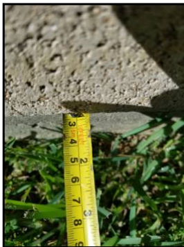
Right side, brick overhangs brick ledge by 1"
