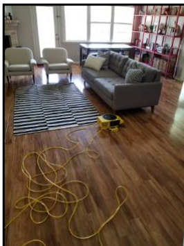
Zip level placed approximately center of house
