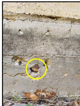
Front corners, brick overhangs brick ledge by 1.5"
