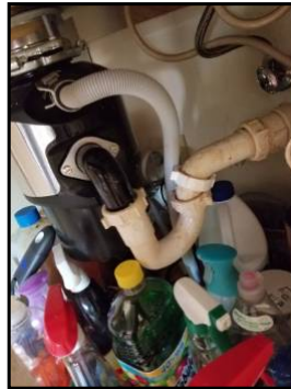
No high loop and/or air gap
