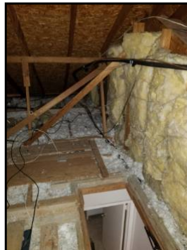
Insulation blown-in and bat
