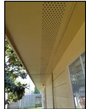
Rear, soffit vent
