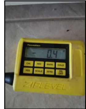
North wall (between master bathroom sinks), -0.4
