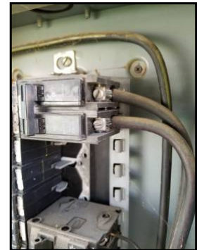
Aluminum 2 AWG for main service conductors, no antioxidant grease present
