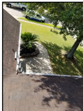
Front middle, gutters with guards installed
