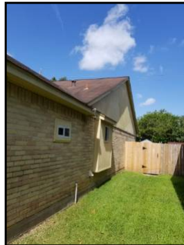
No soffit(except rear) and/or gable vents observed around structure
