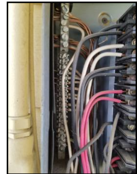
Aluminum 2 AWG for main service conductors, no antioxidant grease present
