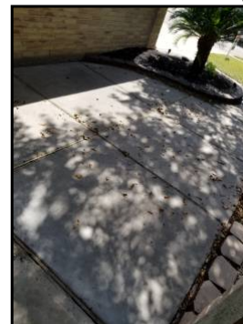
Front patio area, not original construction
