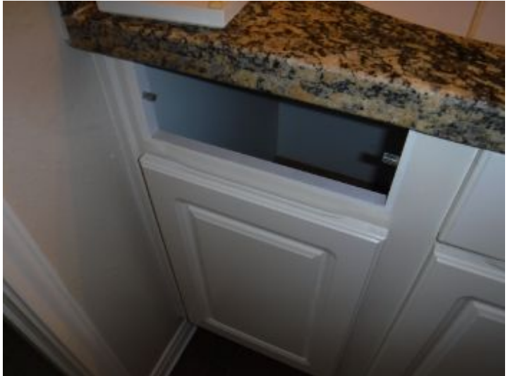
Upstairs bath - Missing tub stopper, broken clip front facing decorative board on sink cabinet and recommend replacing inside parts in commode tank
