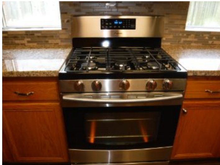
No anti-tilt device bracket on unit
