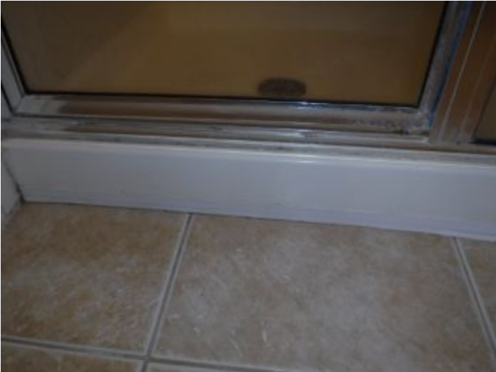
Master bath - Missing bottom seal on shower door
