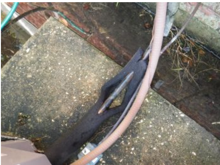
Insulate exterior return line
