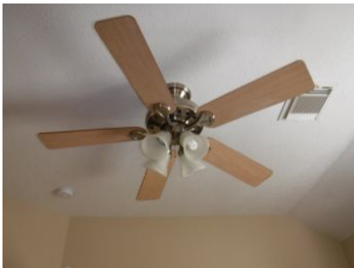
Ceiling fan and light fixture and/or bulb did not function in front bedroom
