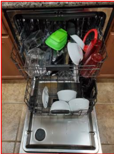
The dishwasher was not properly secured to the cabinetry
