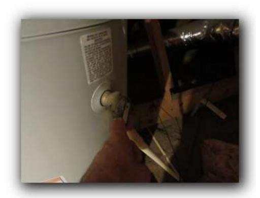
• Corrosion and/or signs of an intermittent leak at isolation valve and/or plumbing connections; IN NEED OF REPAIRS BY ALICENSED PLUMBER.
