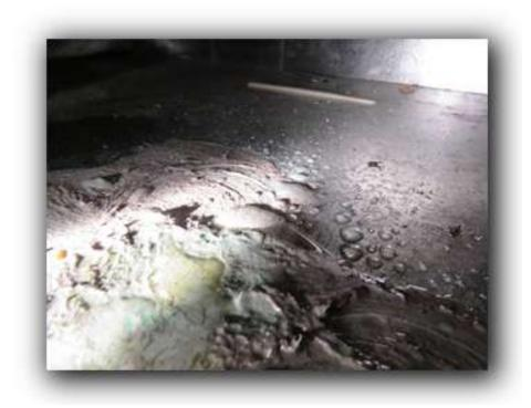
☑ Air handler plenum is not properly sealed;needs evaluation and needs to be properly taped and sealed by a licensed hvac professional.
