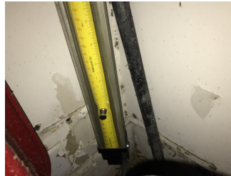
Front right corner at the garage, level with the reference point.
