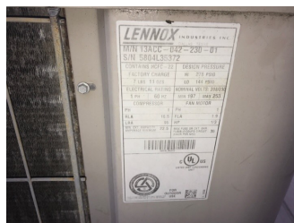
3.5 ton unit, made in 2004 by Lennox, uses R22 coolant, 22.5 35 amp breaker required
