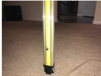
Reference point near the middle of the foundation.
