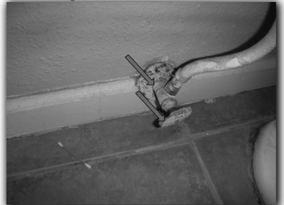
Corrosion / Damaged Handle
