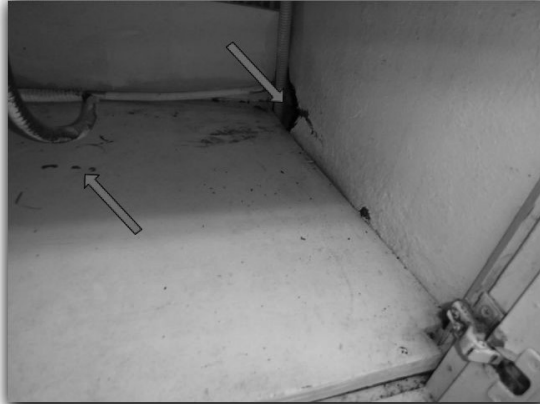
Previous Moisture Damage
