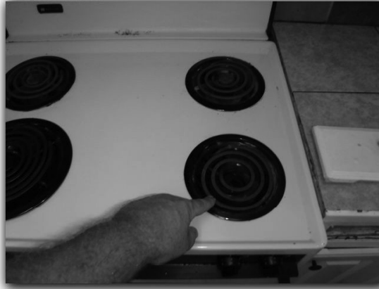
Missing Coil Stand
