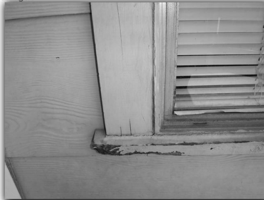
Damaged Glazing
