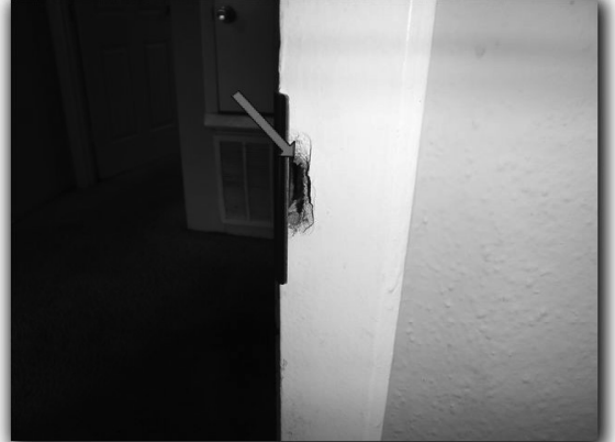
Damaged Stop
