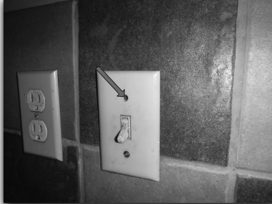
Broken Terminal @ Ground
