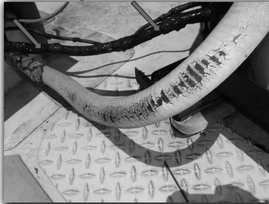
Deteriorated / Missing Insulation
