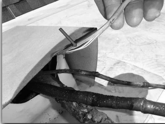
Exposed Wiring
