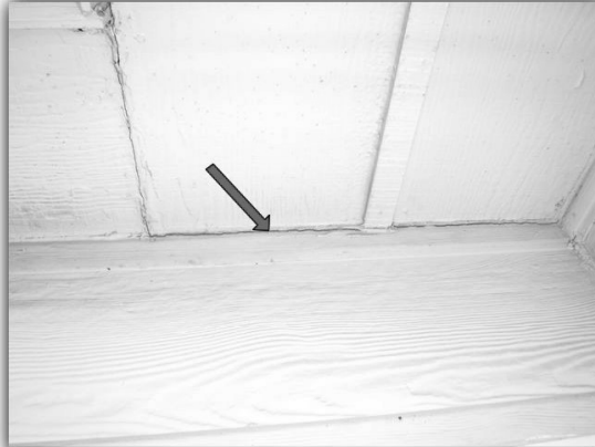
Moisture Damage / Seal
