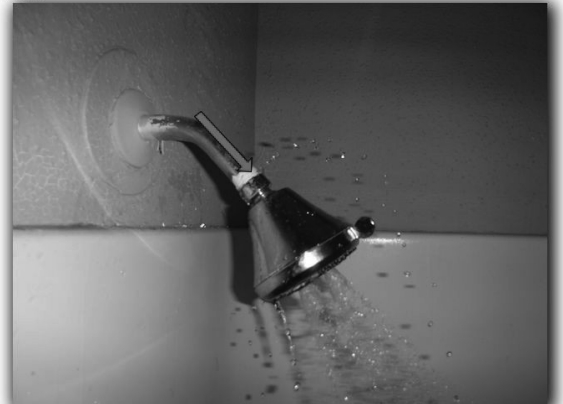
Corrosion / Damaged Handle
