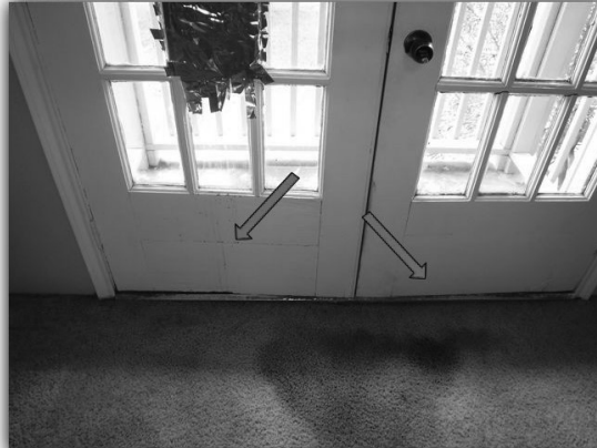
Missing Weather Stripping
