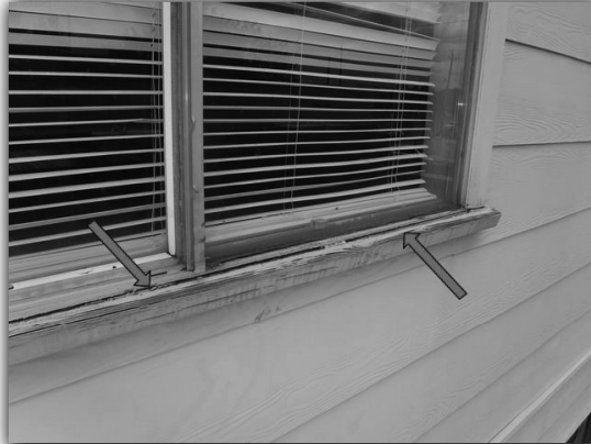
Moisture Damage / Seal
