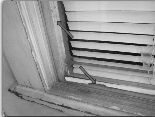
Damaged Glazing
