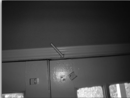
Missing Weather Stripping
