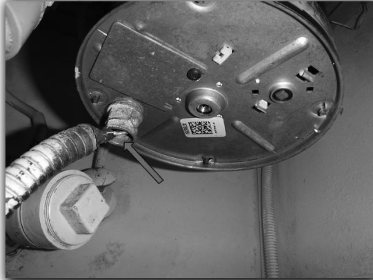
Exposed Wiring
