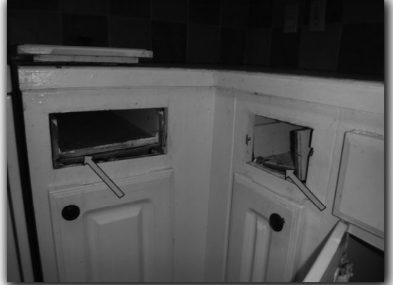
Damaged Drawer Slide
