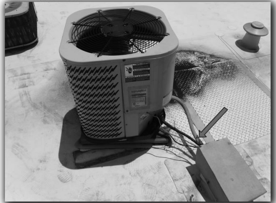
Deteriorated Conduit
