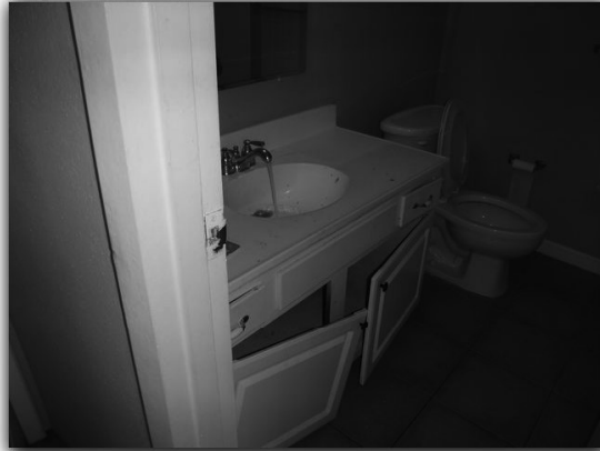
Damaged Door Fronts
