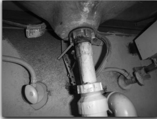
Corrosion @ Drain Connection
