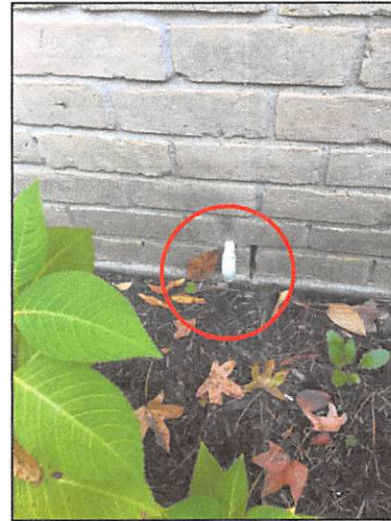
The water heater TPR valve discharge line terminated on the right side of the home
