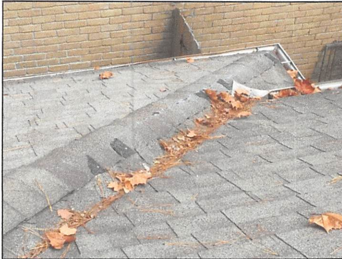
Observed deteriorated ridge shingles
