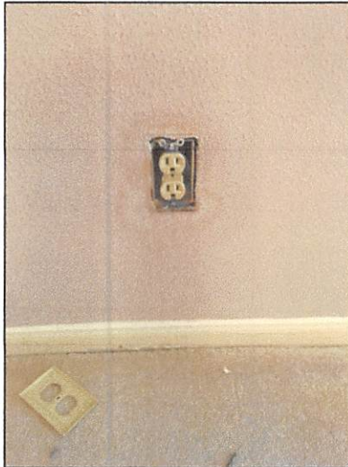
Observed a dry stain on the right wall of the back bedroom
