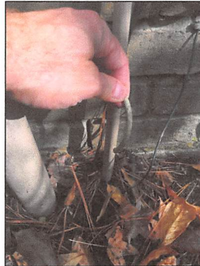
The grounding electrode conductor was disconnected from the exterior grounding rod clamp
