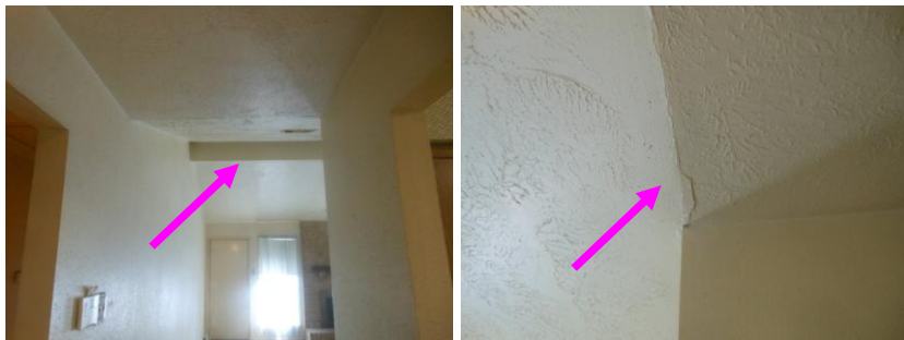
4. Cracked/separated ceiling; at hallway leading to in living room
