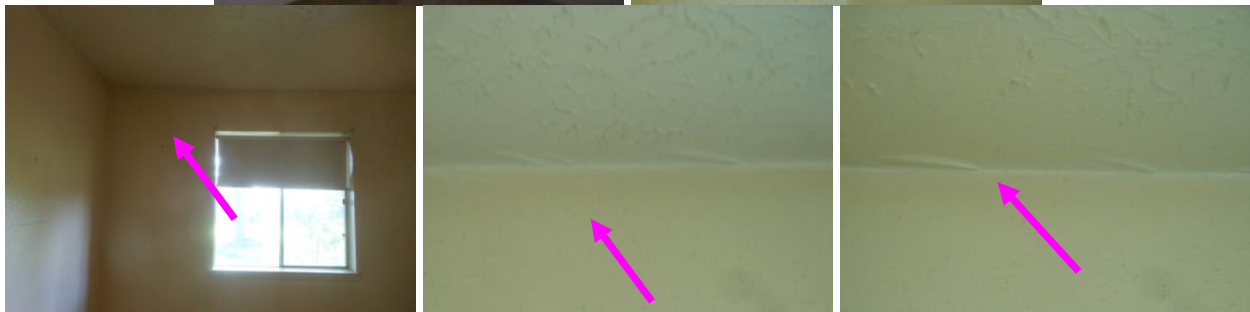
4. Cracked/separated ceiling; at hallway leading to in living room
