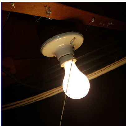
B. Item 9(Picture) attic
