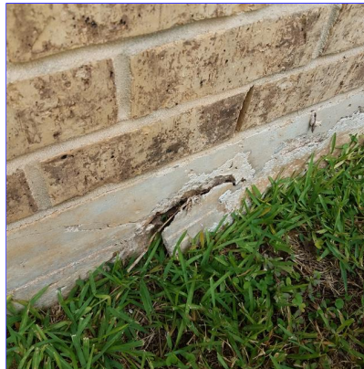
A. Item 4(Picture) left side of garage
