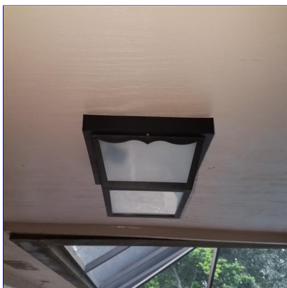
B. Item 12(Picture) back porch
