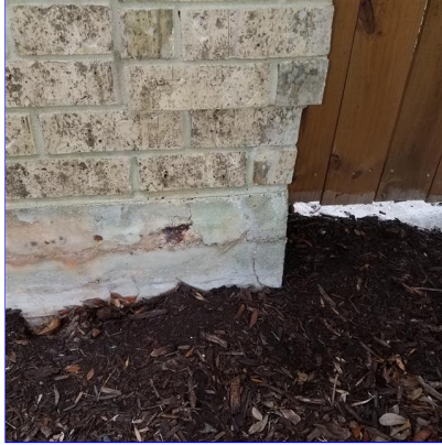
A. Item 6(Picture) front right of home
