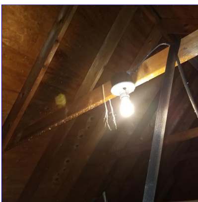
B. Item 8(Picture) attic
