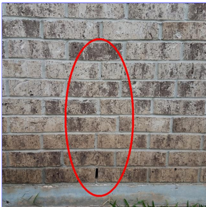
E. Item 3(Picture) left side of garage
