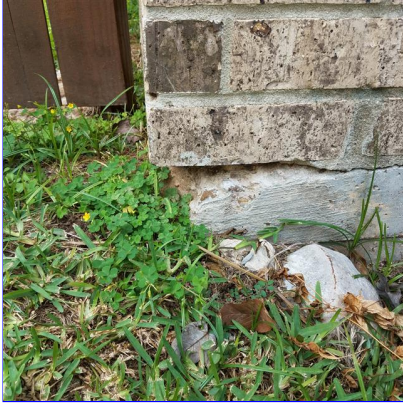
A. Item 5(Picture) left side of garage
