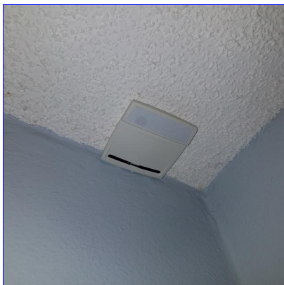
B. Item 10(Picture) master bedroom
