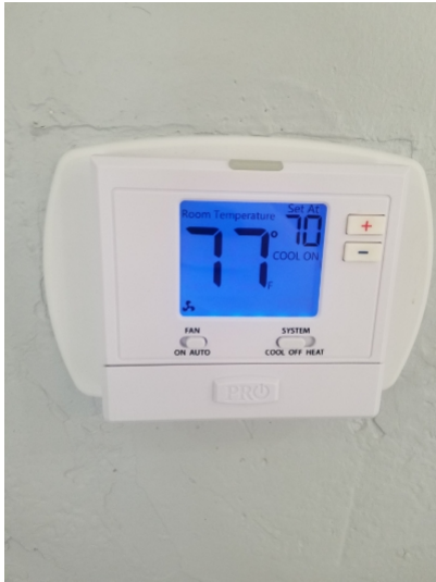
Thermostats were Pro1, digital programmable types.
