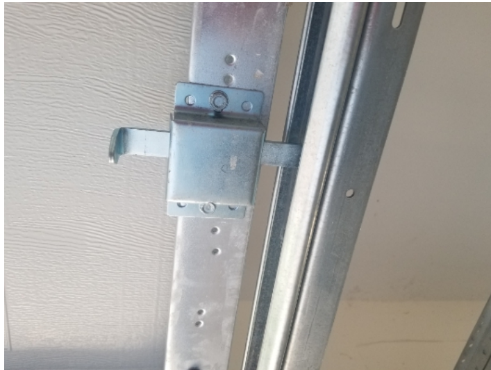
Door lock should be disabled since opener is present.
