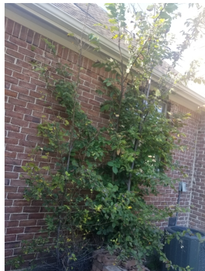
Excessive vegetation was noted in some areas of the home. In our opinion vegetation should be cleared at least 12" from the exterior walls.
