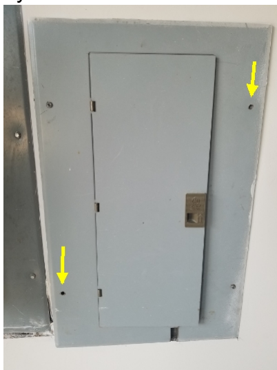
Some fasteners were missing for the panel covers.
