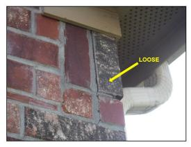
Potential pest / rodent entry; west roof-wall intersection.
