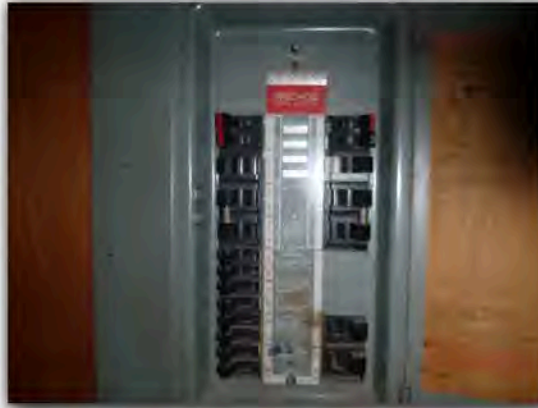
Improper clearance and/or access to panel.
