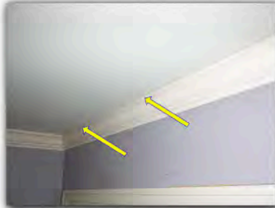
Previous patching and current fractures noted on ceiling in Master bedroom and left rear Bedroom.
