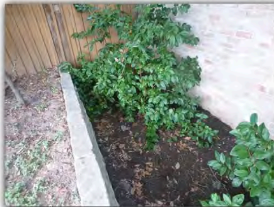
Brick siding improperly installed into grade level around perimeter of house. This limits viewing of base of siding and may allow undetected pest infestation. Newer installations require siding to terminate and drain above soil line.
