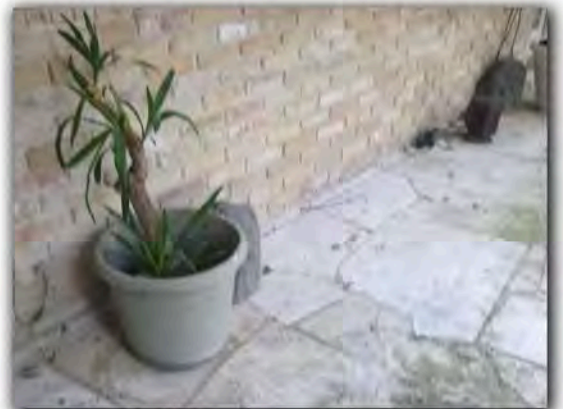
Brick siding improperly installed into grade level around perimeter of house. This limits viewing of base of siding and may allow undetected pest infestation. Newer installations require siding to terminate and drain above soil line.
