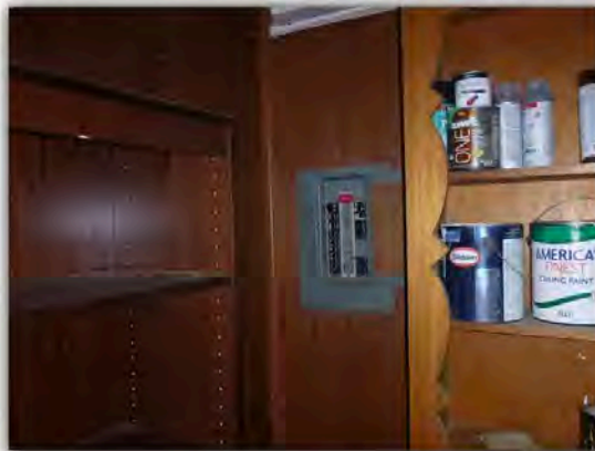
Improper clearance and/or access to panel.
