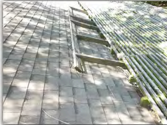
Back patio arbor construction is not properly secured.
