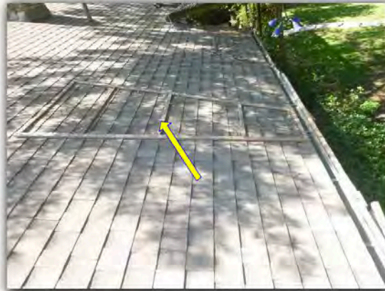
Back patio arbor construction is not properly secured.
