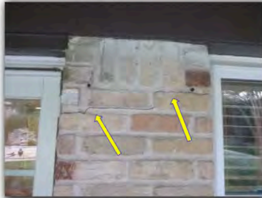
Brick/mortar crack at rear.
