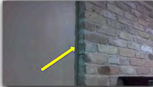
Fracture/separation at wall to fireplace joint. Repair.
