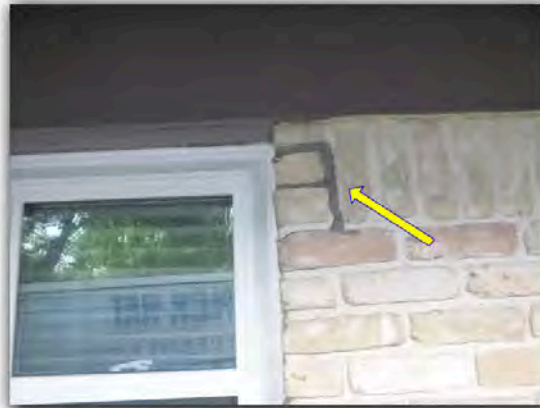
Brick/mortar crack at rear.
