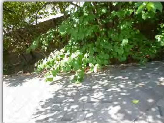
Tree limbs are observed in contact and rubbing the surface of the roof. Trim to avoid excessive wear.
