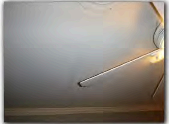
Previous patching and current fractures noted on ceiling in Master bedroom and left rear Bedroom.
