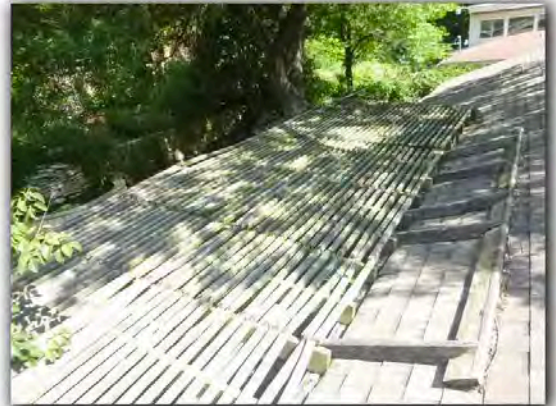
Tree limbs are observed in contact and rubbing the surface of the roof. Trim to avoid excessive wear.
