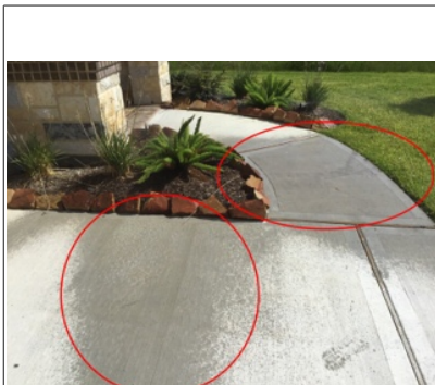
DEFICIENCY: Not all spray-heads work on zone #1 and the one that do work need adjusting.
