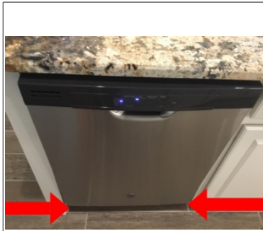
DEFICIENCY: The dishwasher is not secured at the bottom
