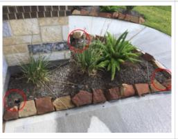
**DEFICIENCY:** Not all spray-heads work on zone #1 and the one that do work need adjusting. Recommend repair by a licensed contractor.
