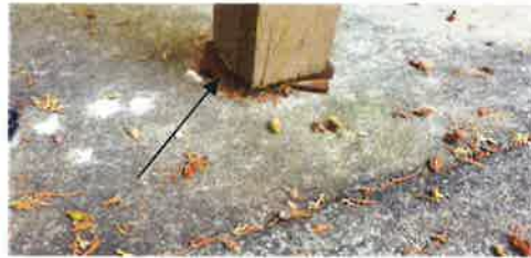
Porch wood structural support posts are not secure properly at base
