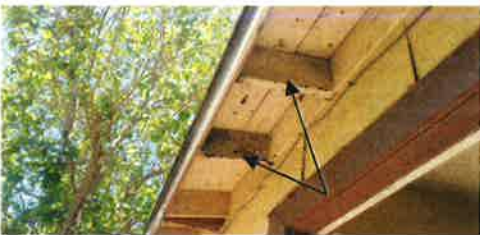
Several rafter tail ends are rotted at rear cornice
