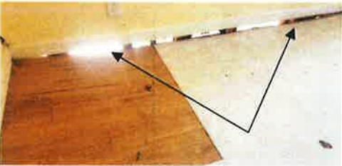
Floor surface has fallen in at rear right dining room
