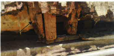
Siding base areas are open at rear exposing rotted wall studs and bottom plate
