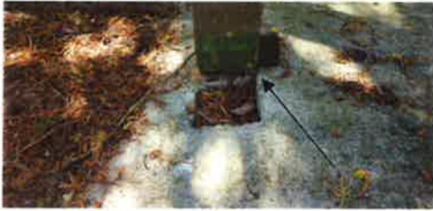
Porch wood structural support posts are not secure properly at base
