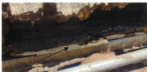
Siding base areas are open at rear exposing rotted wall studs and bottom plate
