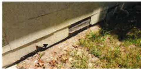
Siding base areas are open at rear exposing rotted wall studs and bottom plate
