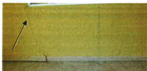
There are vertical wall corner and wall – ceiling taped joint cracks as several locations
