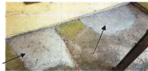
Foundation was previously repaired evidenced by patched concrete repair holes at the front porch and rear patio
