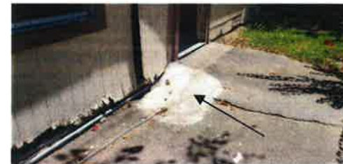
Foundation was previously repaired evidenced by patched concrete repair holes at the front porch and rear patio
