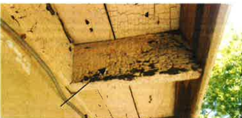
Several rafter tail ends are rotted at rear cornice
