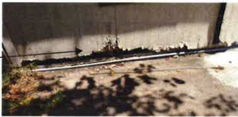
Siding base areas are open at rear exposing rotted wall studs and bottom plate
