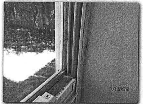
X: The interior walls at the Master bedroom windows have organic growth. Possible water intrusion at the windows.
