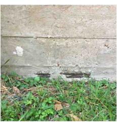
• Hairline cracks were noted in the expose grade beam in a few places. These are considered typical for settling of the structure on these soils. Monitor areas for future performance.
