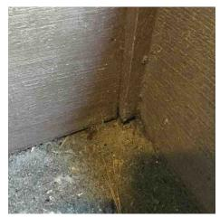
• Repair moisture damage to base of front porch column
