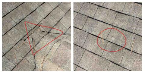
• "Bird-eyes" are apparent where nails have backed out and lifted shingles above. Nails need to be reseated and loose shingles caulked.
