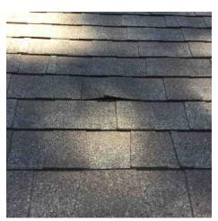
Roof covering appears to be nearing the end of its life expectancy, but appears to be functioning and should be able to be maintained in the short term with monitoring and minor repairs. Covering should be budgeted for replacement in the near future.
